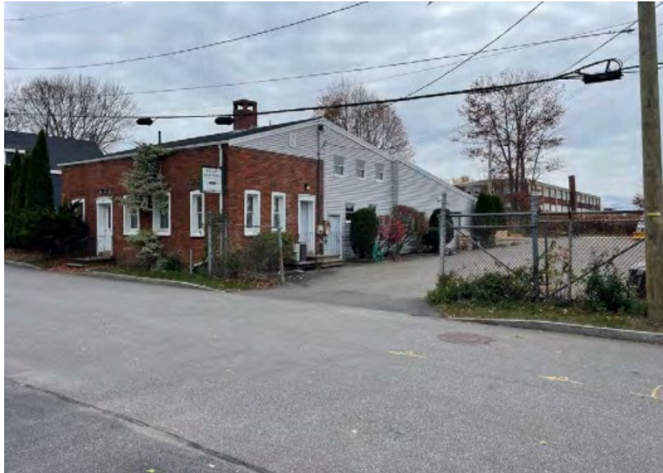
View of Property from Langdon St
