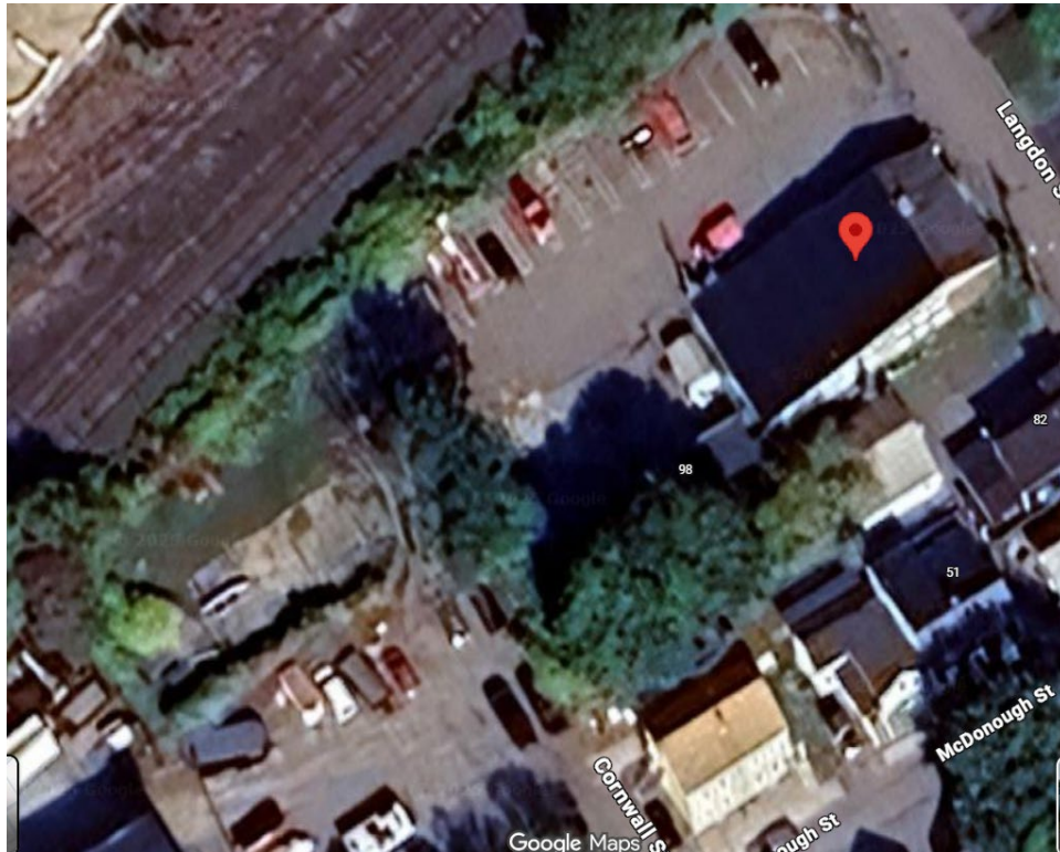
Aerial view of 94 Langdon St & 98 Cornwall St
