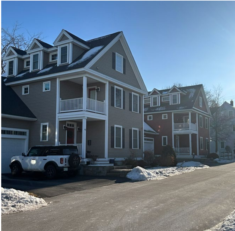
More abutting homes (constructed by Chinburg).
