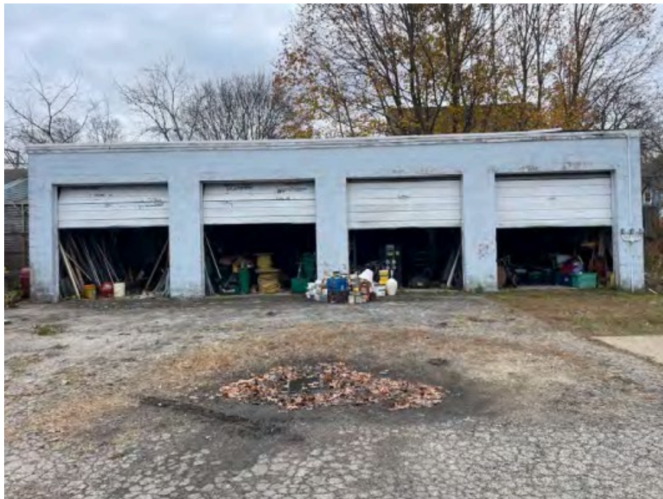
Garage at 98 Cornwall
