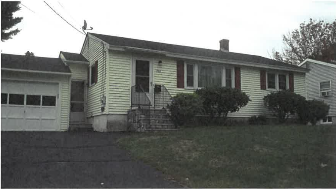
West Elevation looking from Leslie Drive. Garage will be removed and replaced with the proposed addition. New garage will be at the basement level and driveway will be excavated lower.
