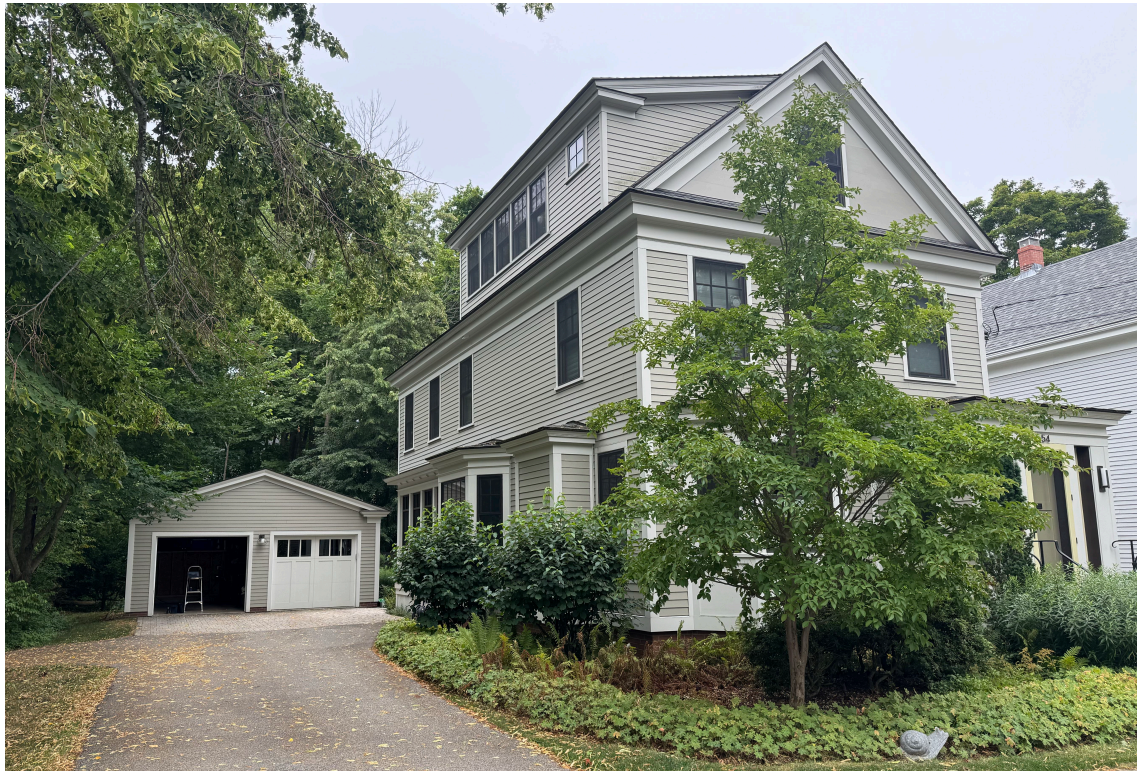
1 EXISTING HOUSE AND GARAGE
