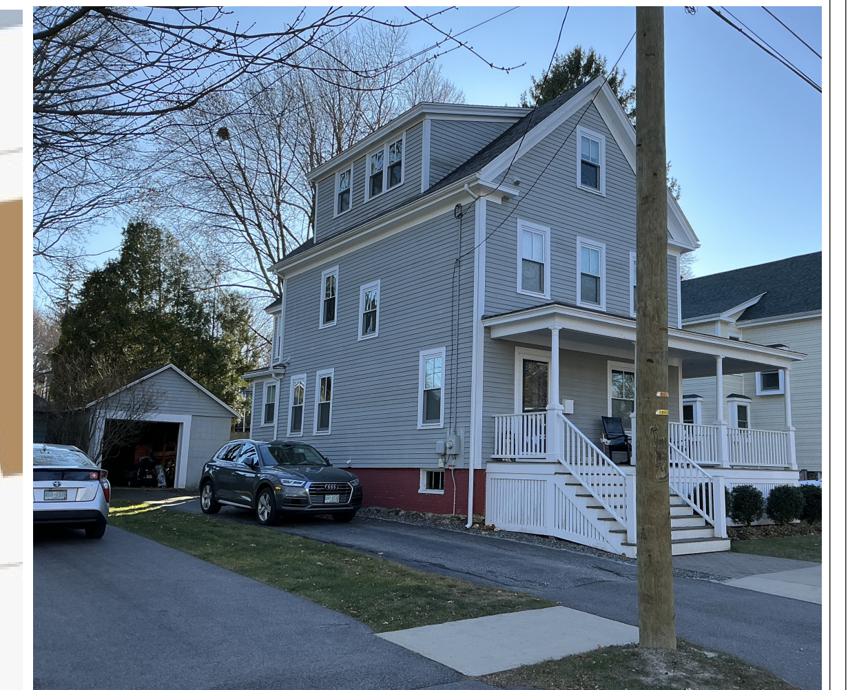
EXISTING CONDITION PHOTO
