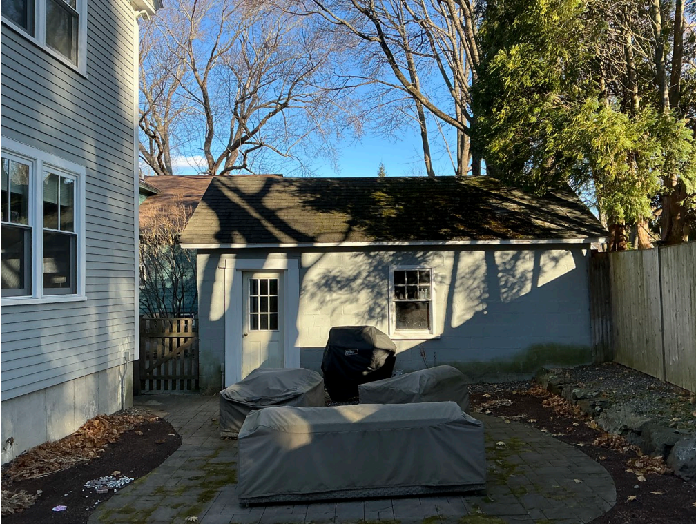
GARAGE RIGHT SIDE:
