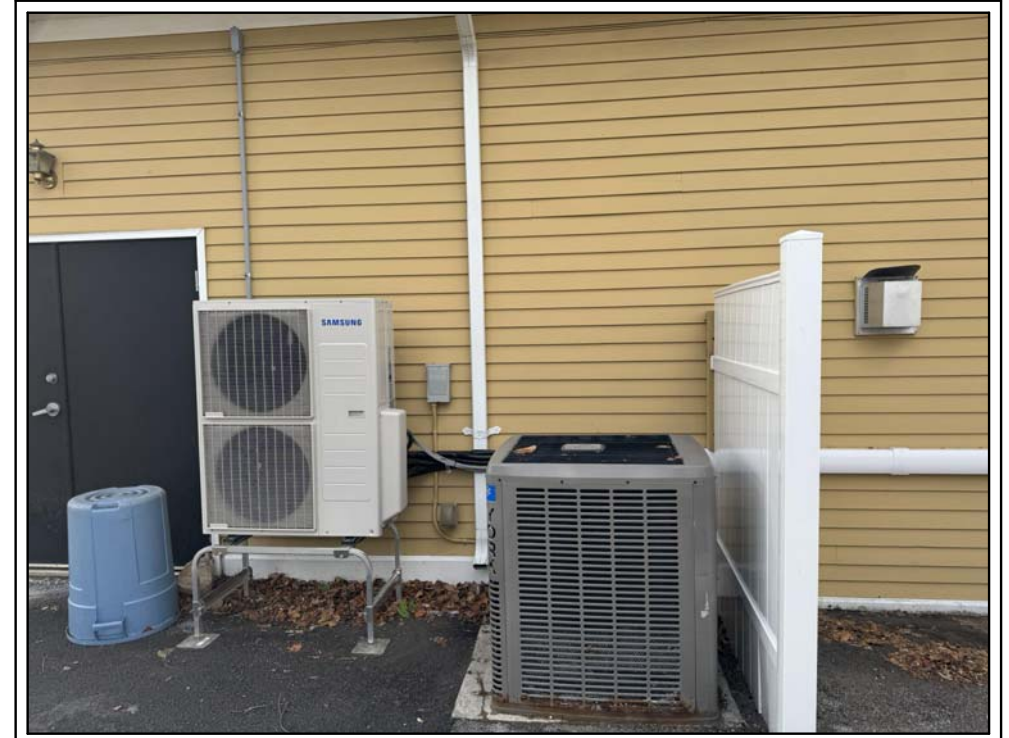
VIEW OF EXISTING UTILITIES AND SERVICES ON WEST SIDE OF BUILDING
