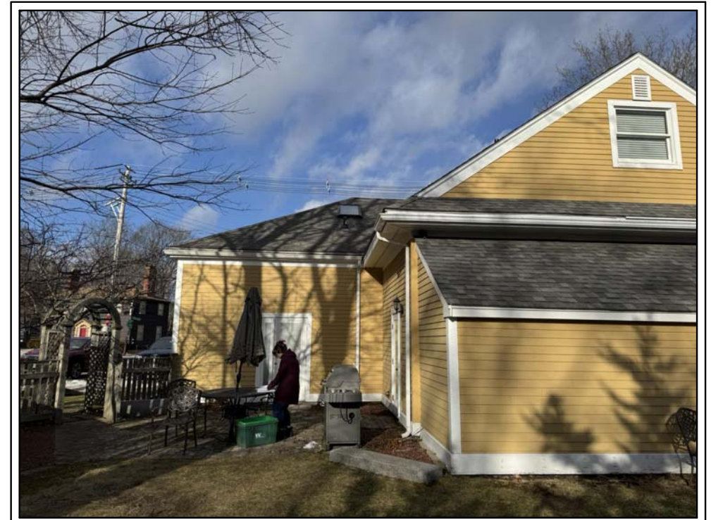
PERSPECTIVE FROM BACK OF BUILDING, SHOWING THE YARD
