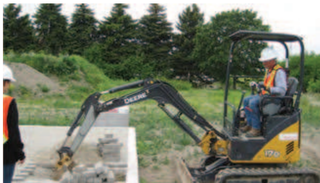
Removal of pavers and granular base.
