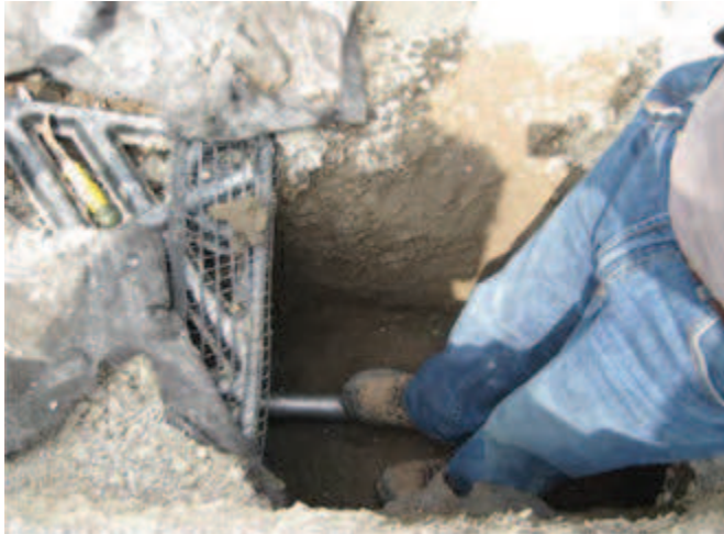
Torpedo set to begin at the imaginary building end of the lateral line.
