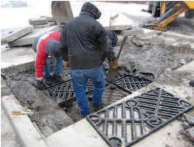
Manual removal of two decks, unscrewed and set aside for future re-installation.
