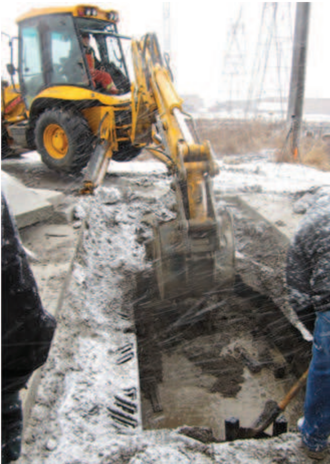
Mechanical removal of soil cells.
