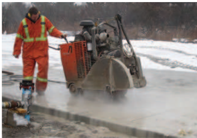
Sawcutting concrete pavement.
