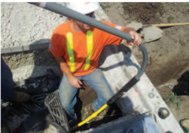
Riser is attached and pulled through.
