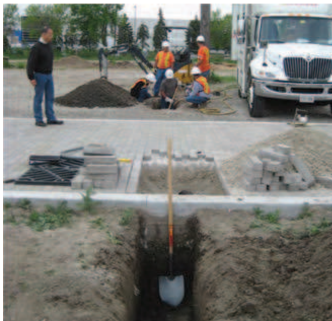
Digging down approximately two cells deep at both lateral ends.
