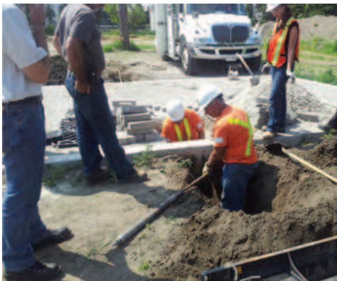
Torpedo and hose are pulled up and out of the pit.
