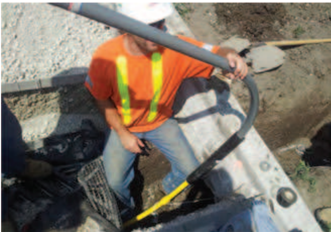
Riser is attached and pulled through.
