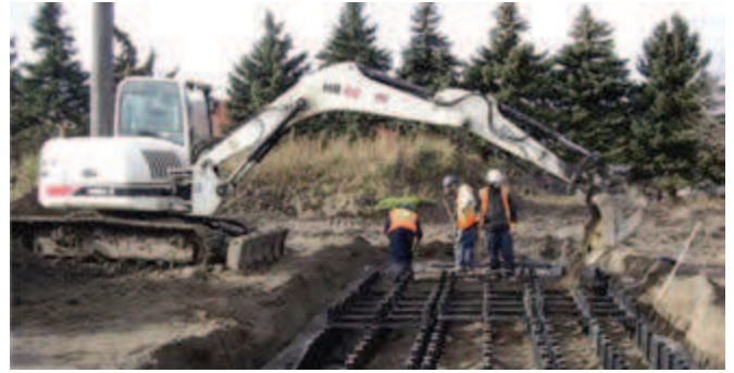
Soil cell trench filled with soil.
