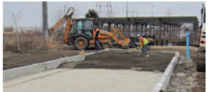
Backfill installation on top of deck.
