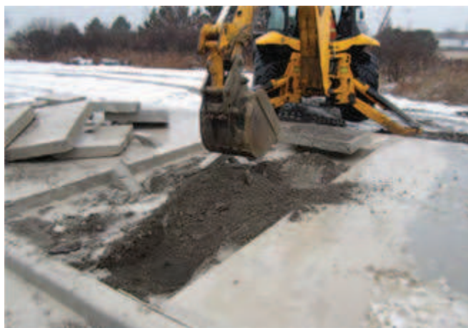
Mechanical removal of pavement to expose soil cell decking system.
