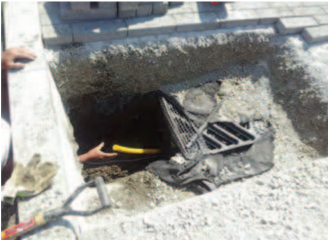
End of lateral at building end.
