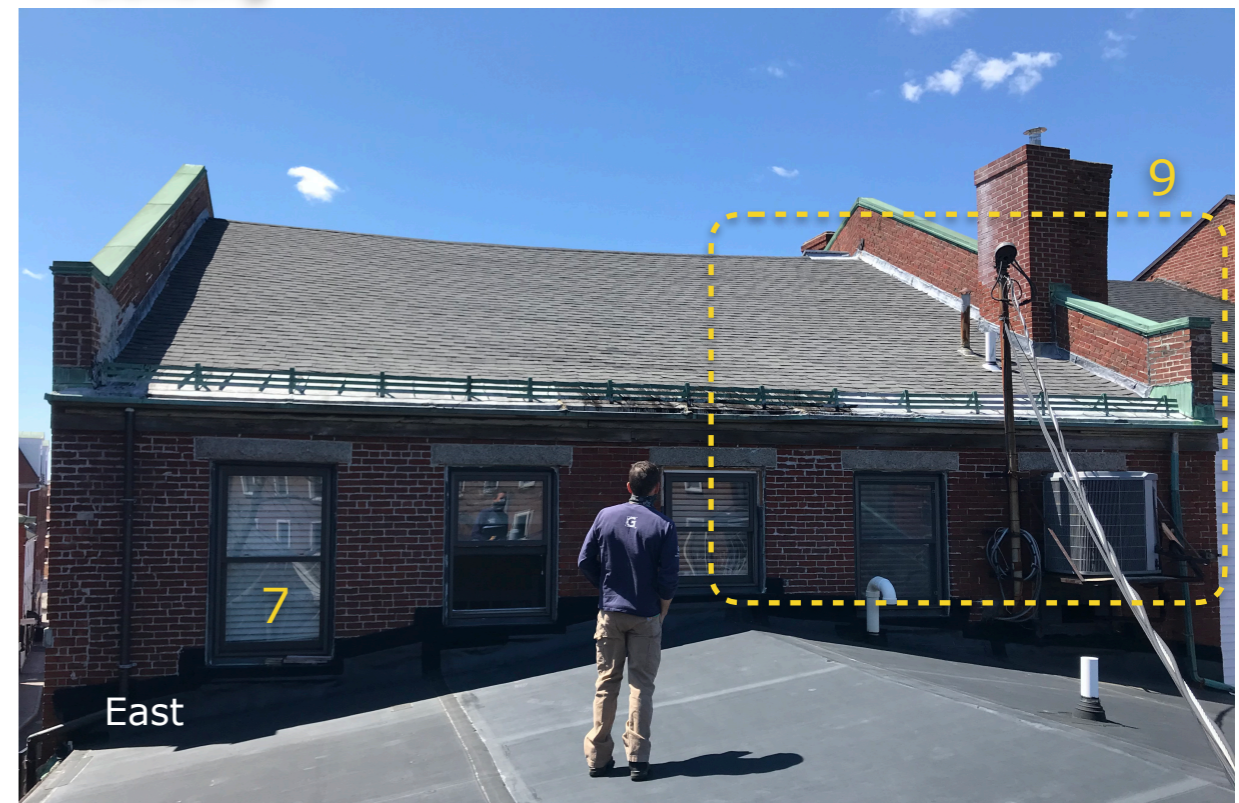
Exterior View at Rear (Above Salt Cellar)
