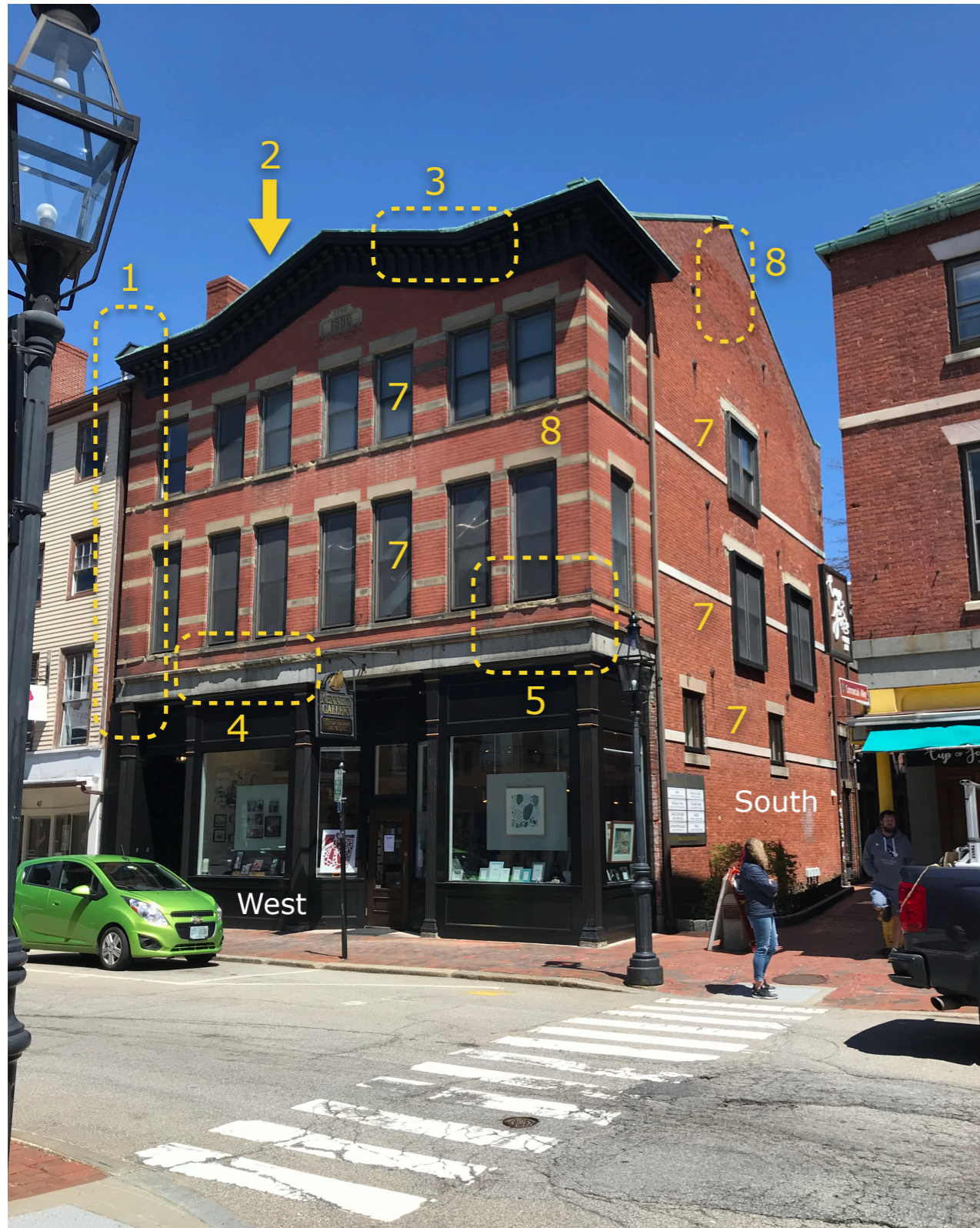
Market Street & Commercial Alley View of Exterior
