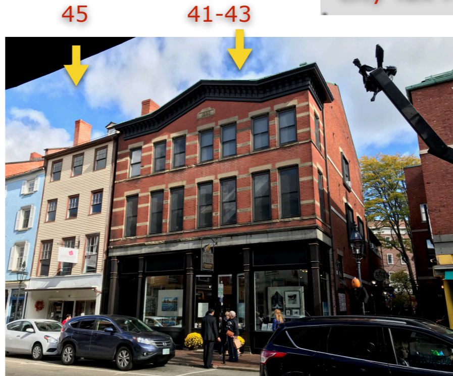
Market Street & Commercial Alley View of Exterior
