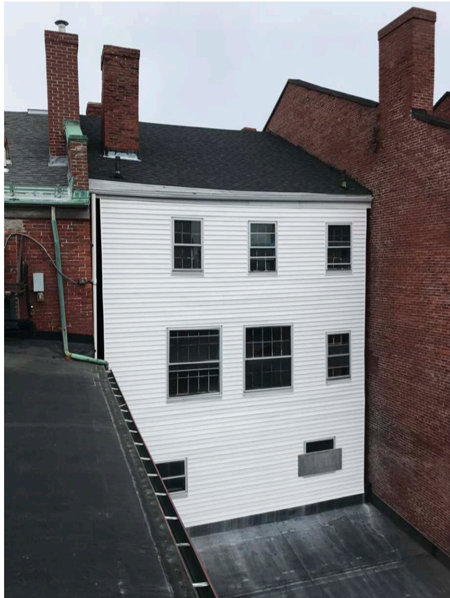
Existing Rear Elevation Photo #1
