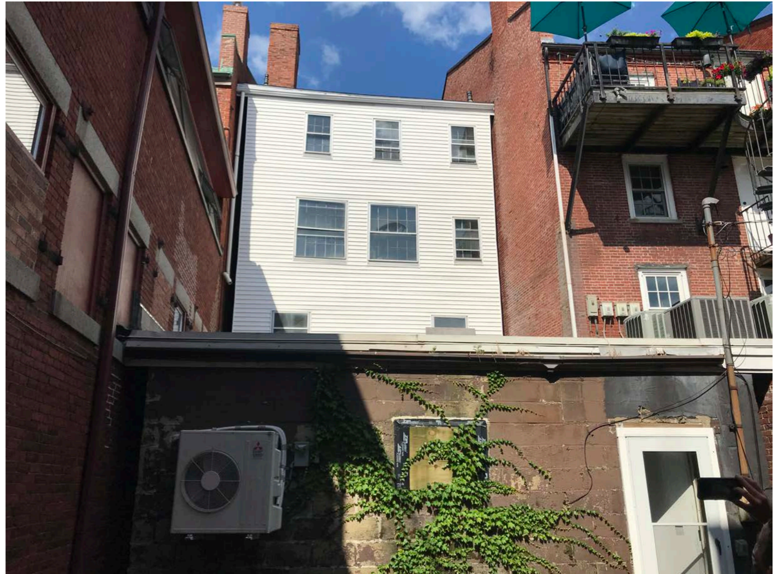
Existing Rear Elevation Photo #2
