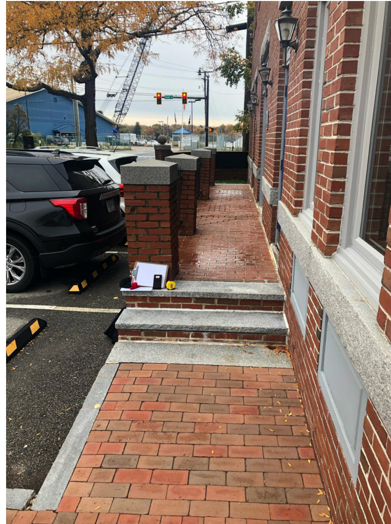
VIEW FROM CURRENT EAST STAIR ENTRY TO EXISTING/CURRENT BUILDING
