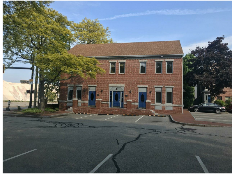
EXISTING/CURRENT SOUTH ELEVATION FROM ACROSS PARKING LOT
