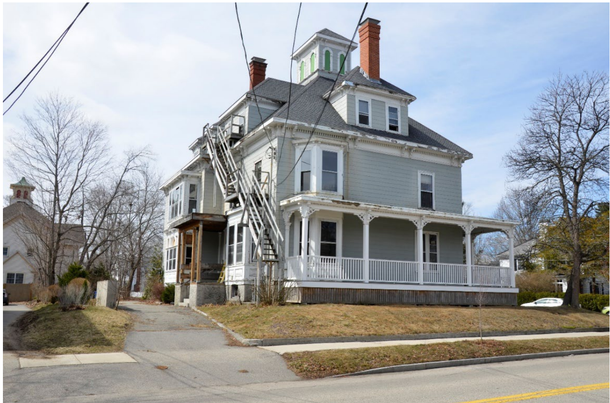
Current view from Miller St. showing the footings for the porte-cochere.
