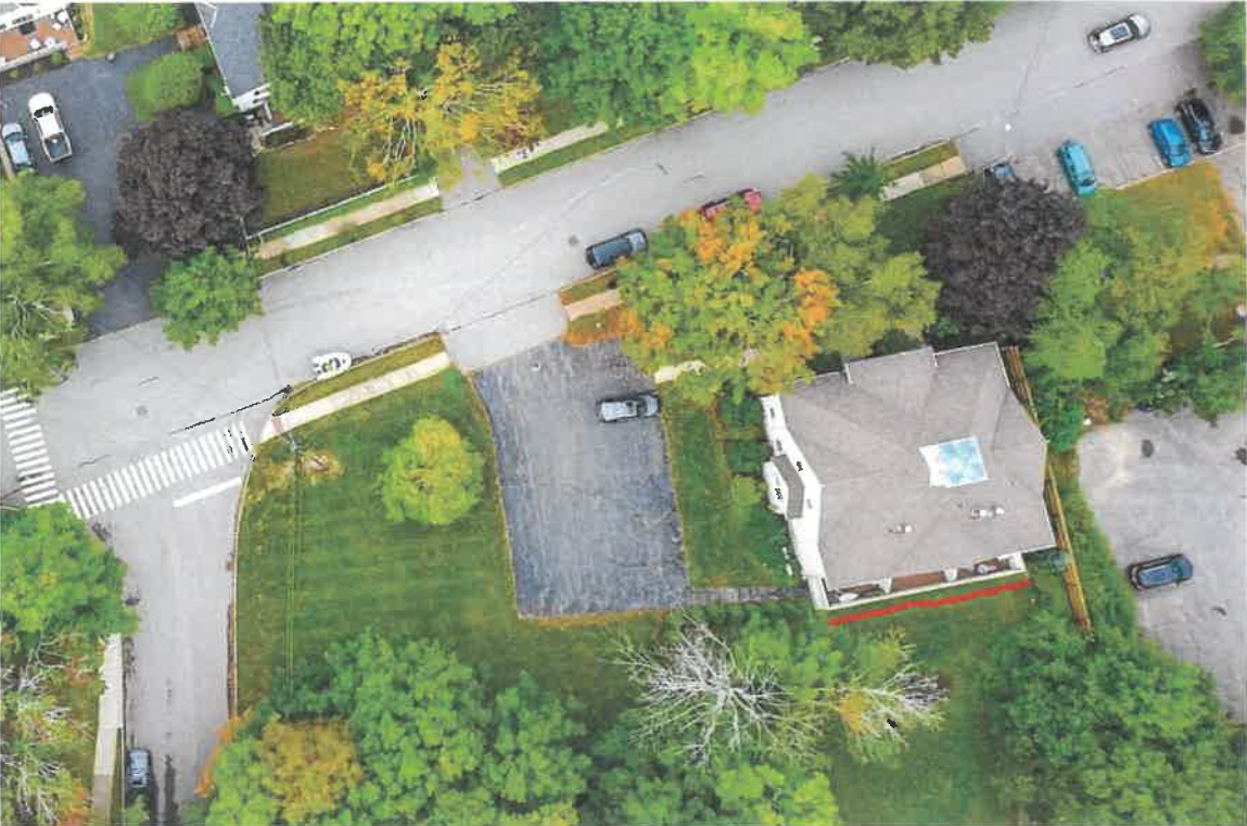
Aerial view of 40 Merrimac Street with proposed 48' x 10' deck on rear of structure (2 additional feet).
