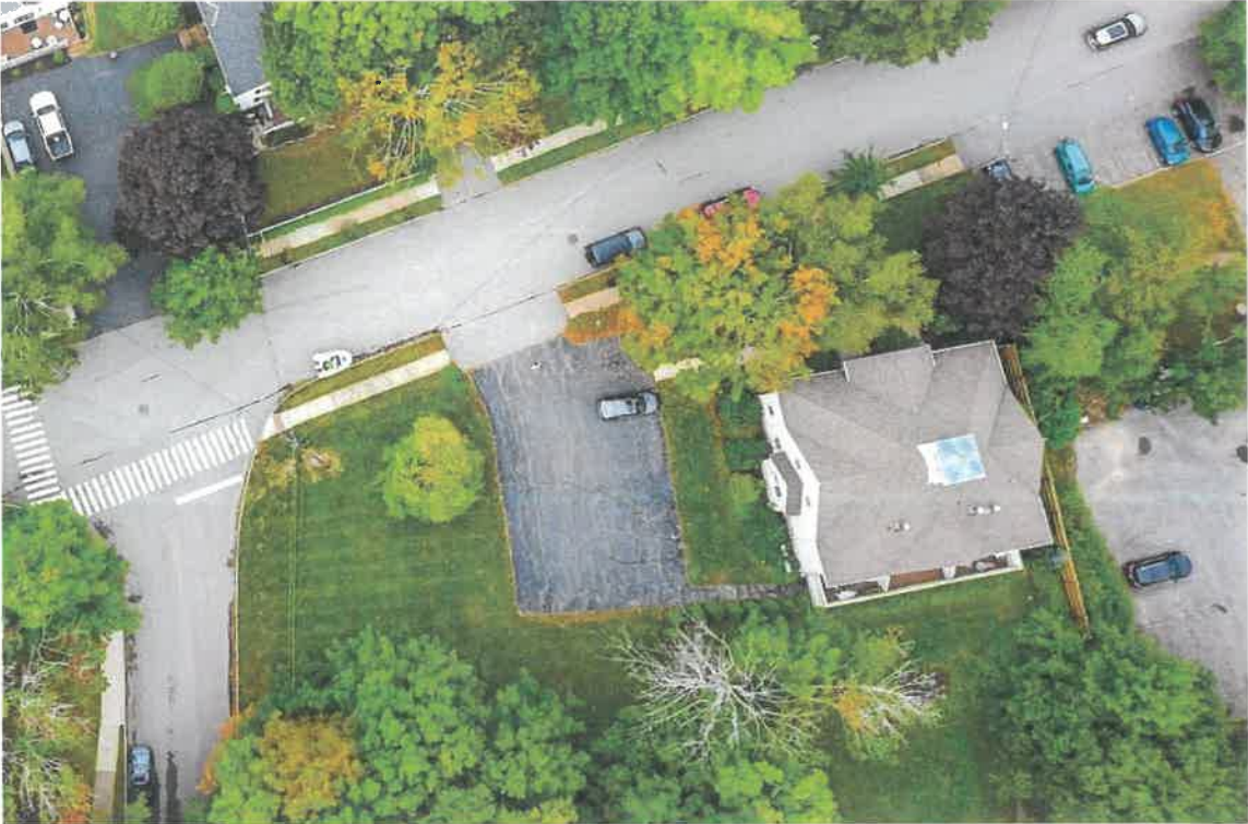
Aerial view of 40 Merrimac Street with existing 48' x 8' deck on rear of structure.
