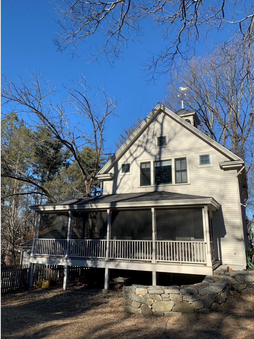
View of Carriage House (Single Family Residence) from rear (west)
