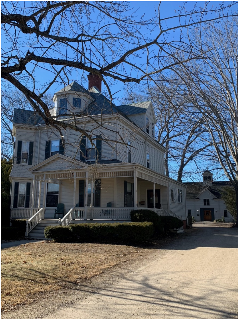
View of existing buildings from Middle Street
