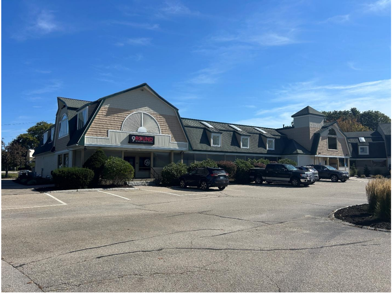
Left Side of Building where Suites 2 and 21/22 are Located
