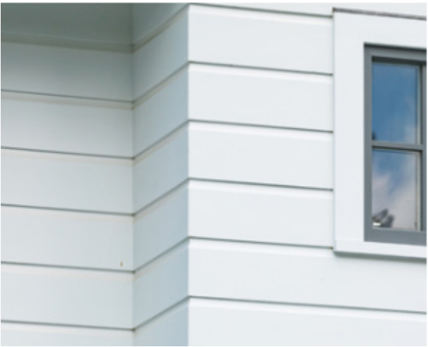
EXAMPLE OF MITERED CORNER IN BORAL
