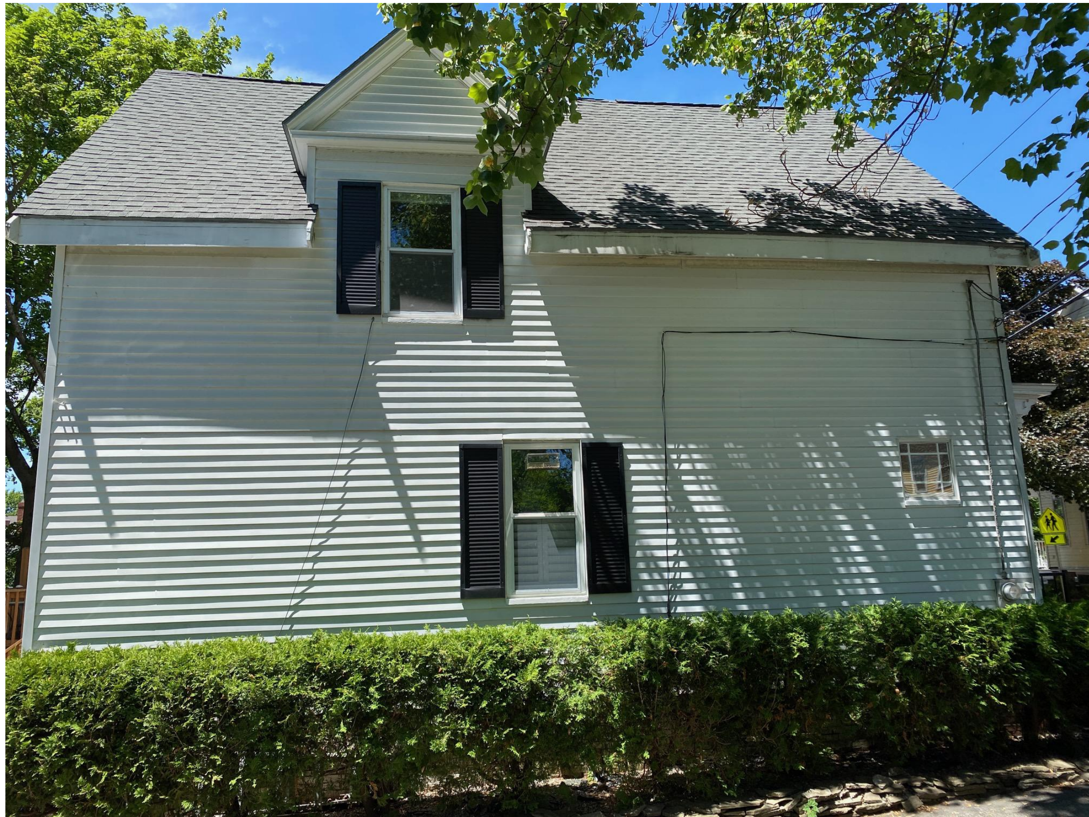
LEFT ELEVATION PHOTO | SIDEVIEW
