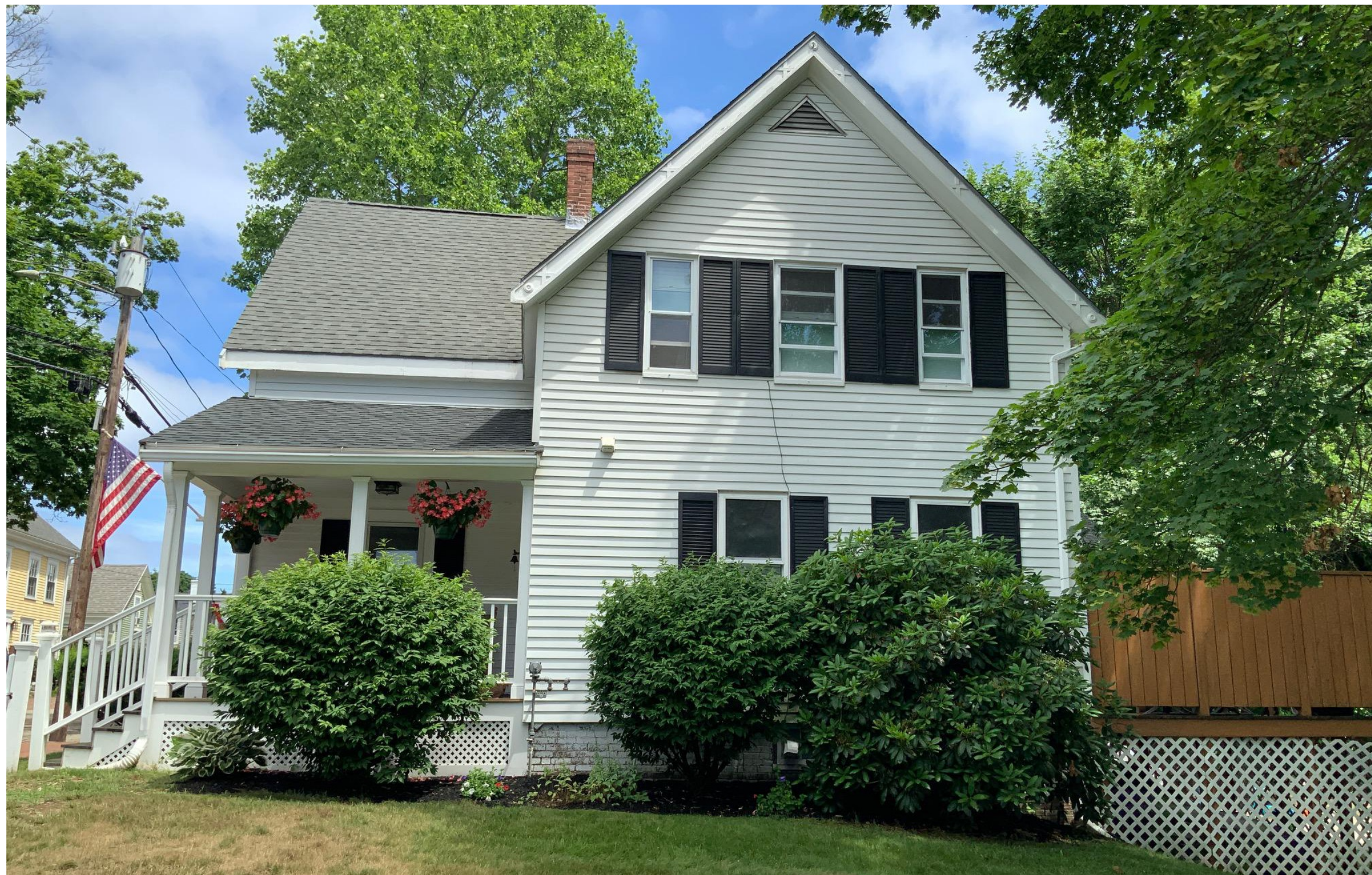
RIGHT ELEVATION PHOTO | SIDEVIEW
