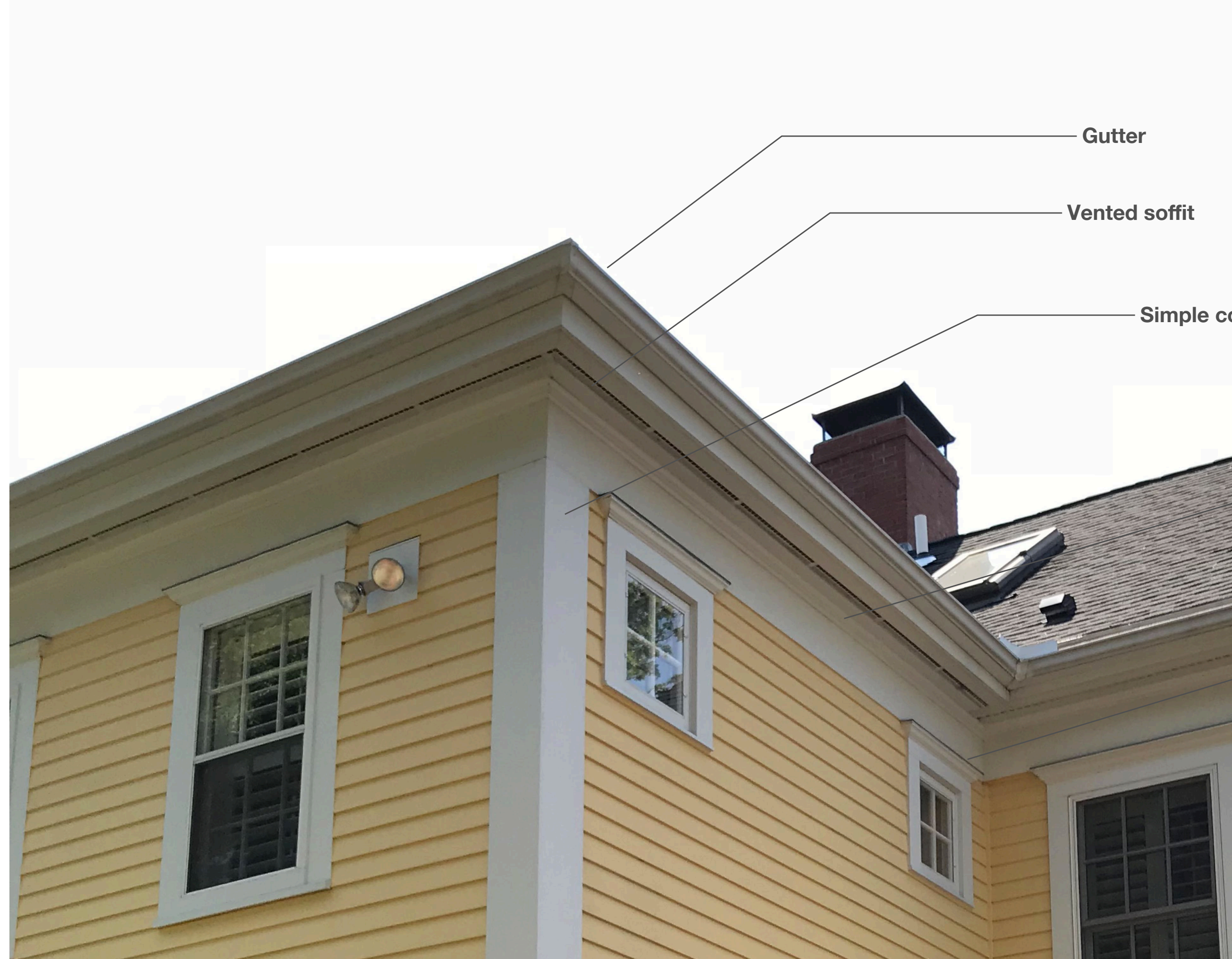
Existing Roof and Trim Detail
