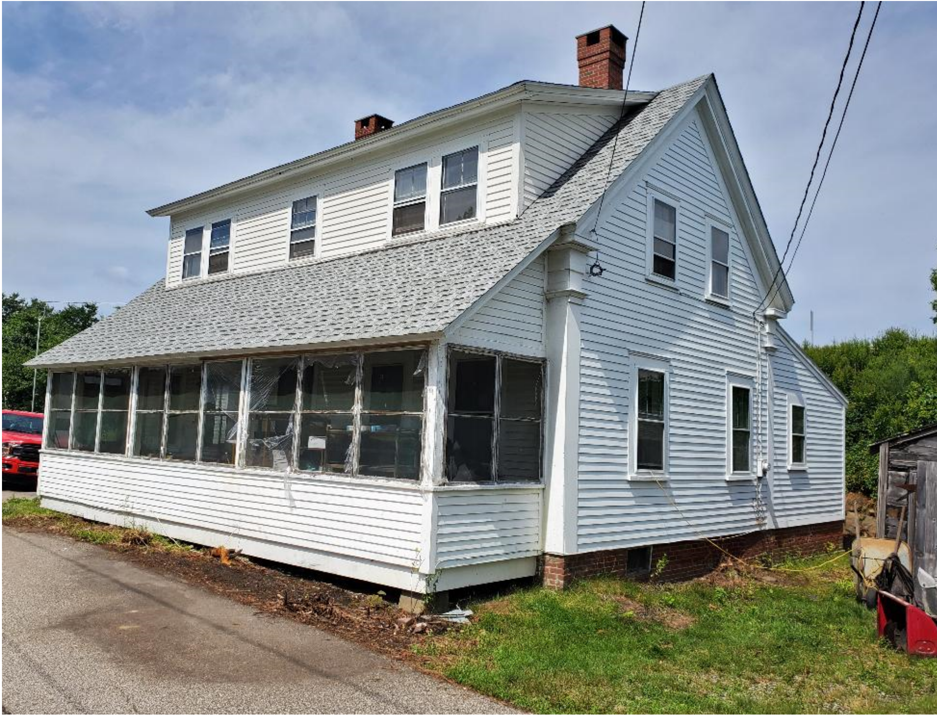
PHOTO- LOOKING AT NORTHWEST CORNER
