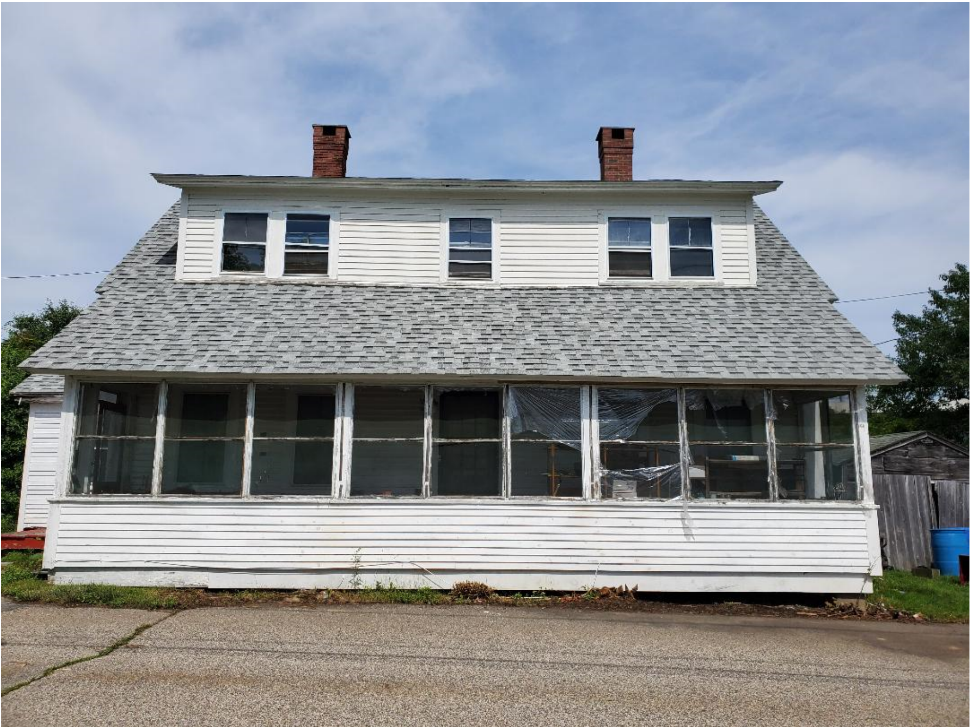
PHOTO- EAST ELEVATION
