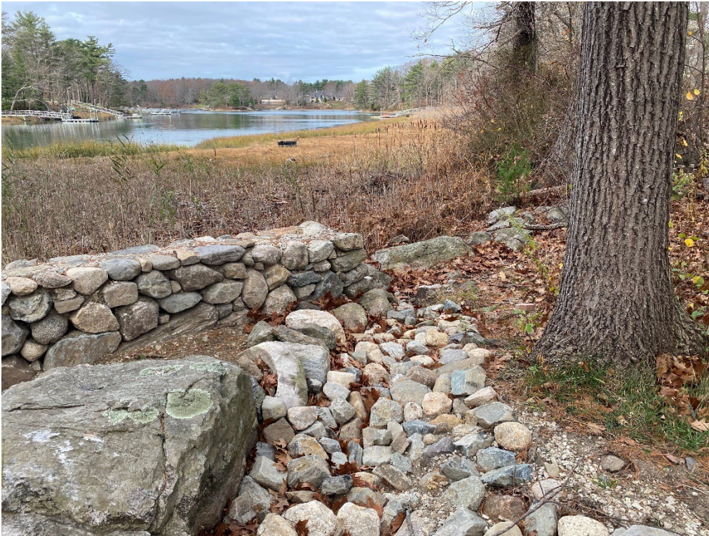
Photo 32. Bottom of the stone swale, viewing northwest. (11-11-22)
