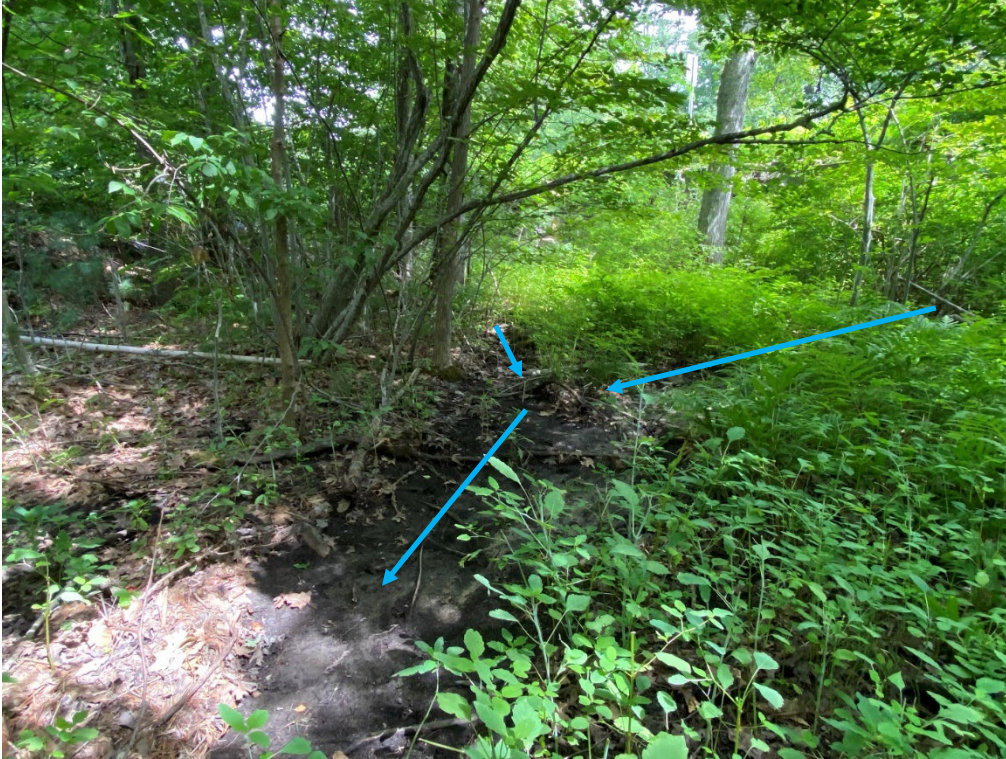
Photo 19. POGS1 leading onto the Gardner property from the culverts located at the northeastern end of POGW2, viewing northeast, upstream. Head wall from which the flows are sourced is in the upper right portion of the photo. Blue arrows indicate the paths of POGS1 and POGS2 from the two culvert outflows from the headwall to where they merge in the foreground. (08-11-22)
