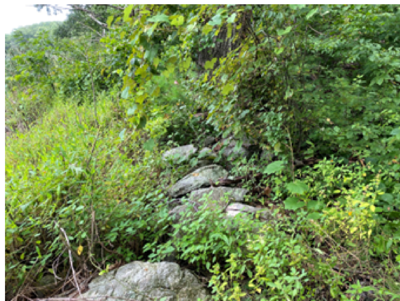
FIGURE 1. UNDISTURBED PORTION OF STONE WALL AT NORTHERN END OF PROPERTY. CORRESPONDS WITH THE SECTION OF STONE WALL CIRCLED IN RED IN FIGURE 2. (8/26/23)
