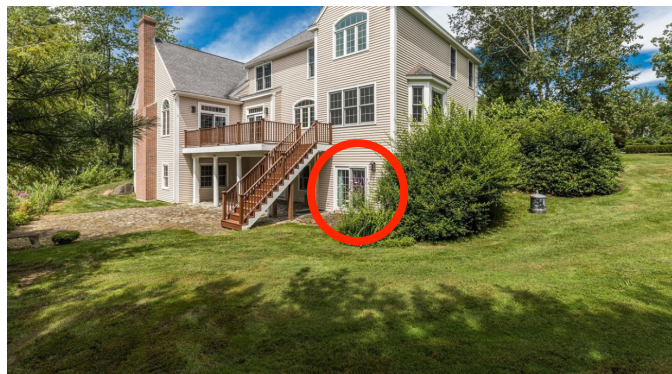
Exhibit #5, Walkout Basement Doorway
