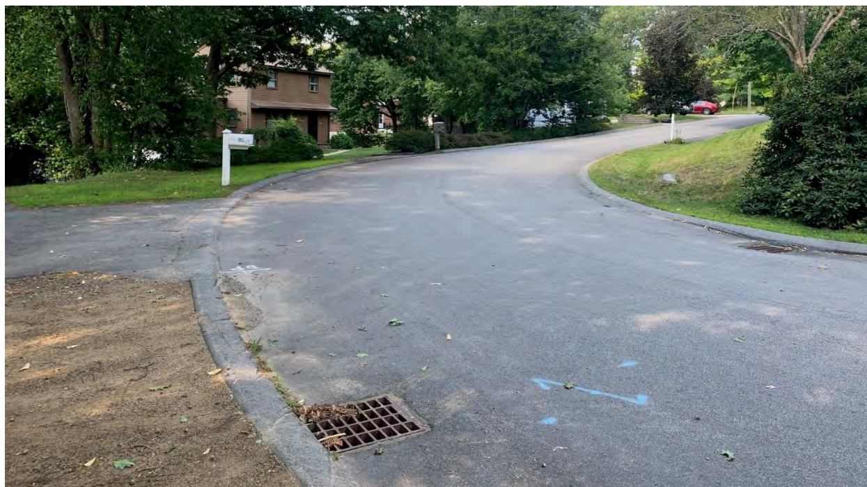
Photo #2: Looking to the North East along Martha Terrace. Taken 8/26/2020.
