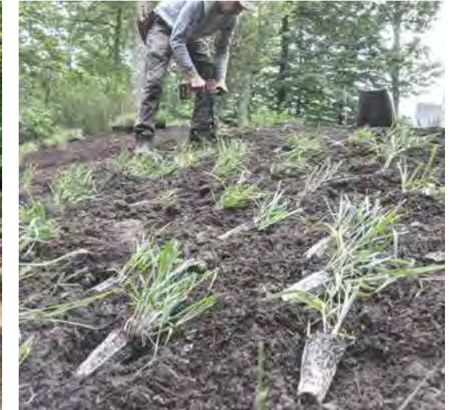
Laying out plugs ensures even vegetated cover.
