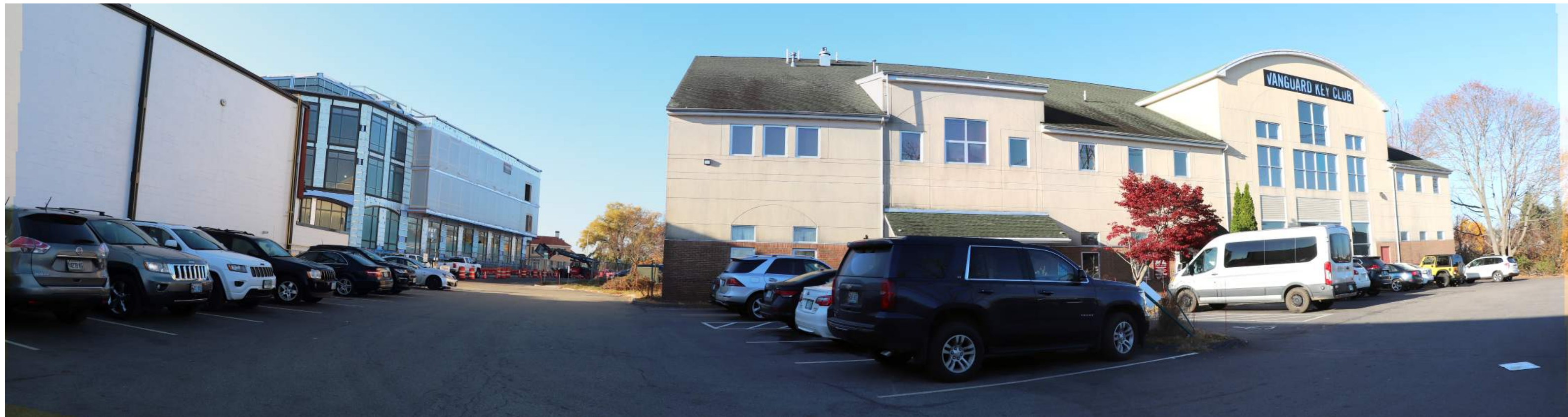
1 1 RAYNES AVENUE FROM PARKING LOT
