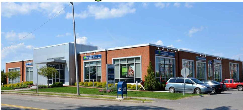
⑤ 111 MAPLEWOOD AVENUE
