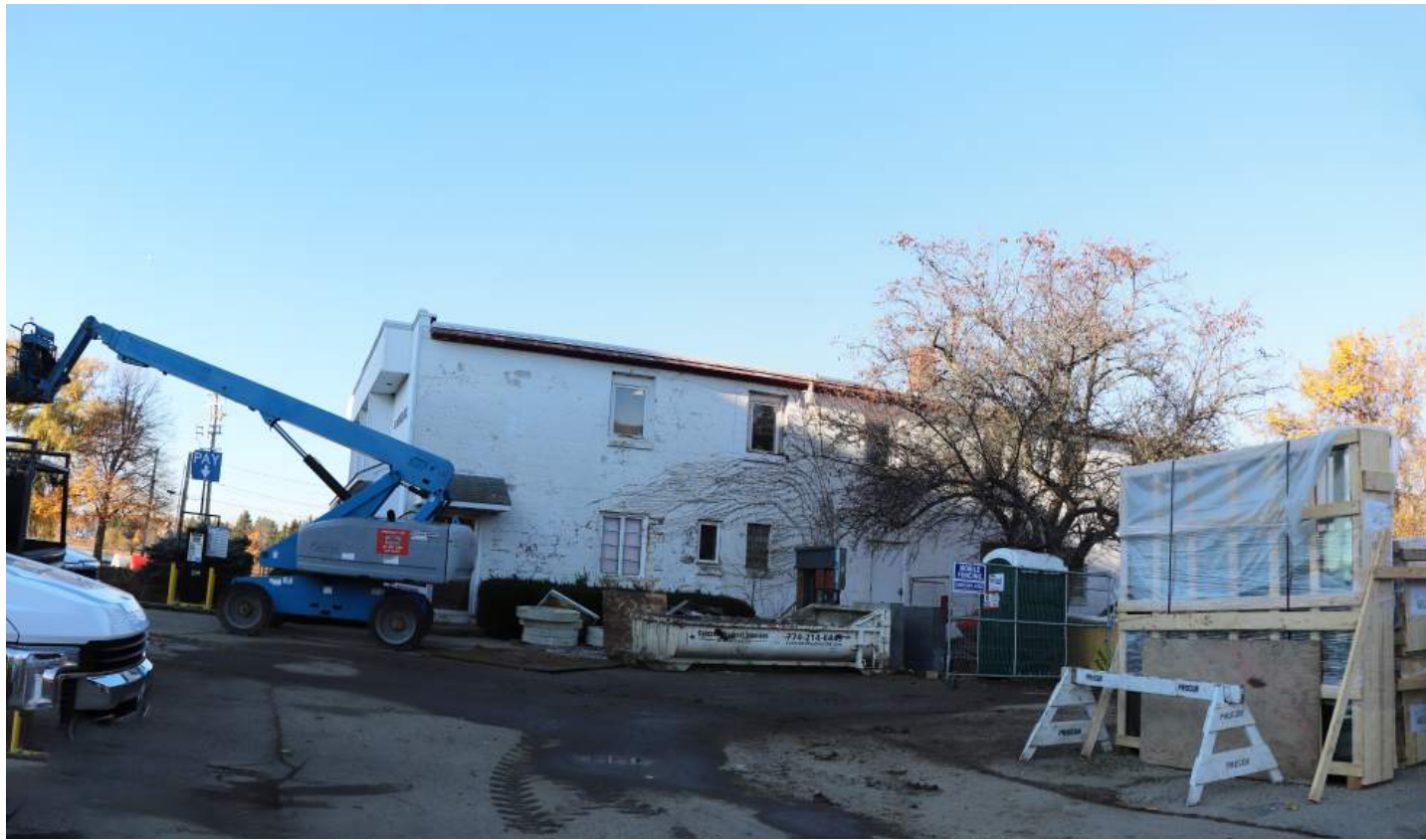
3 31 RAYNES AVENUE FROM PARKING LOT
