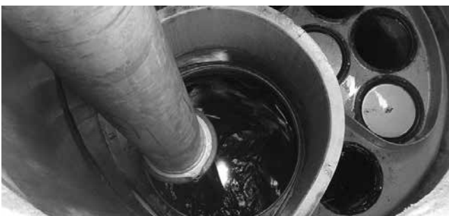
Vacuuming Sump Through MAW
