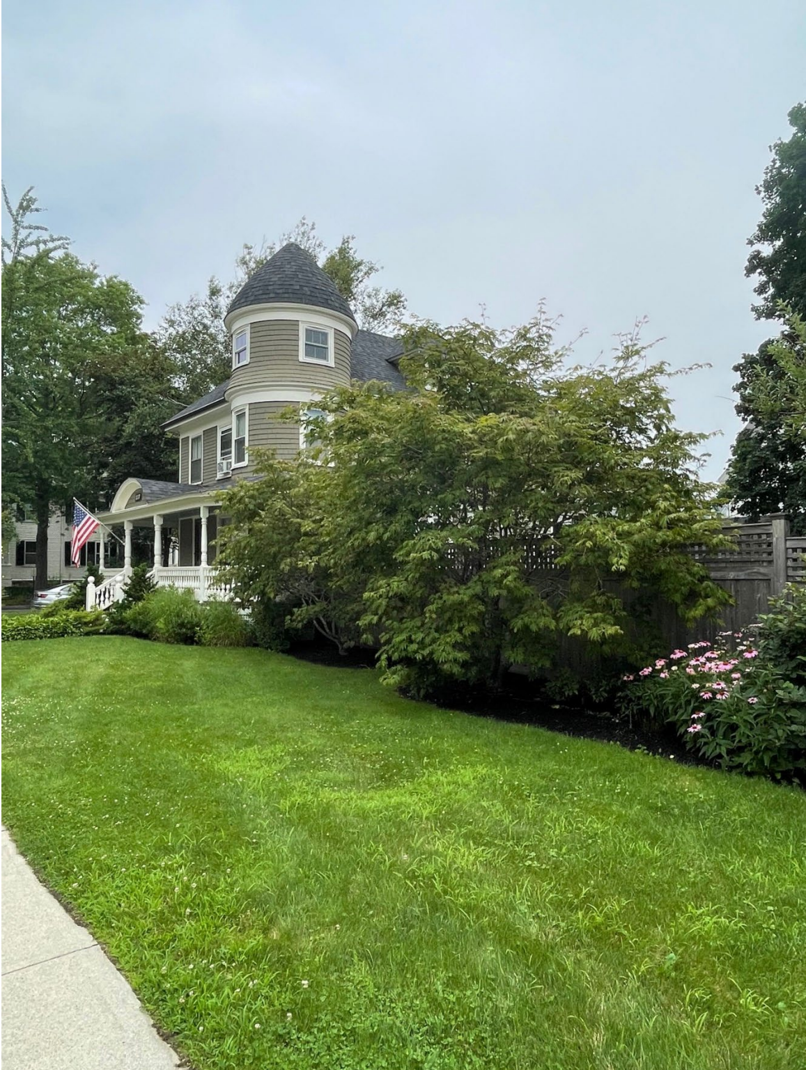
Front Right View of Property (Richards Ave)
