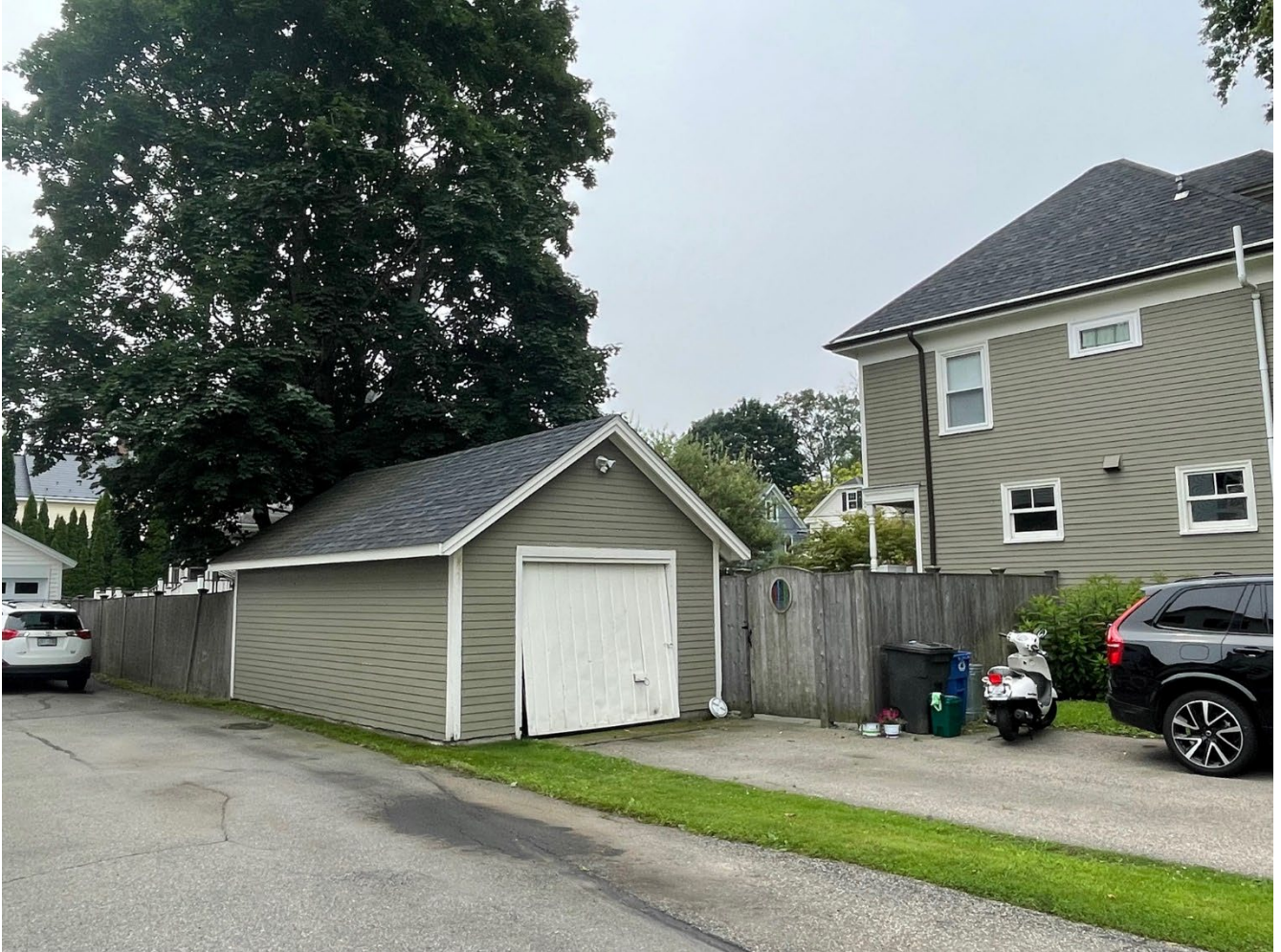
Rear View of Property, Garage & Driveway (Lincoln Ave)
