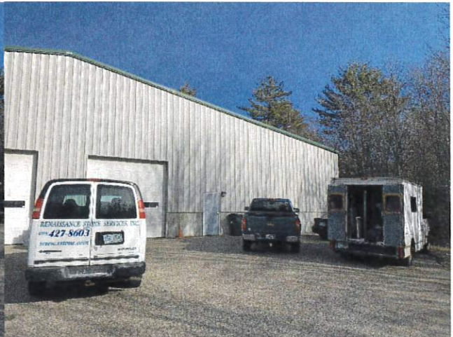
Rear View of 6A Parking Area
