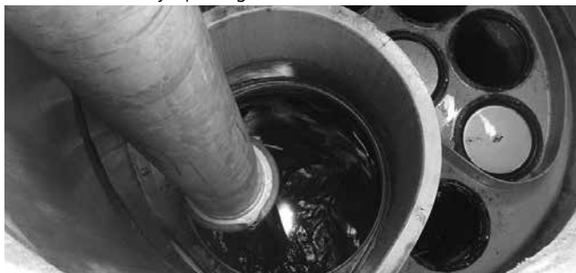
Vacuuming Sump Through MAW
