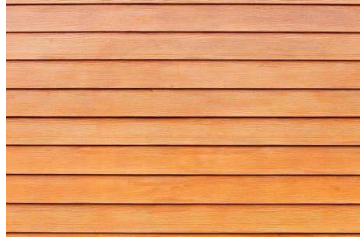
WOOD CLAPBOARD SIDING
