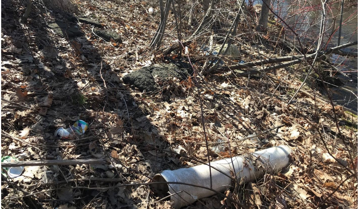
Photo #1: looking at the small debris and larger plastic piping as well as some larger chunks of asphalt on the bank.
