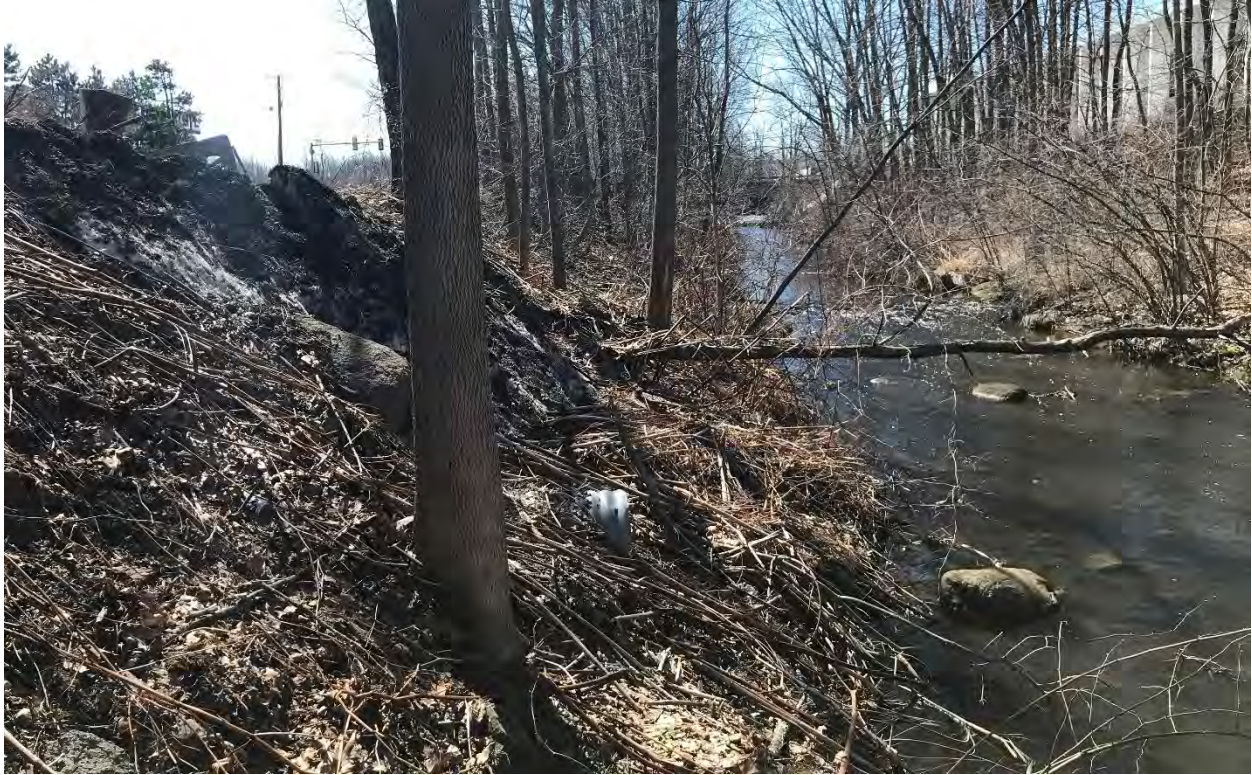
Photo K3: Looking towards Route 1 along the bank at impact area #2
