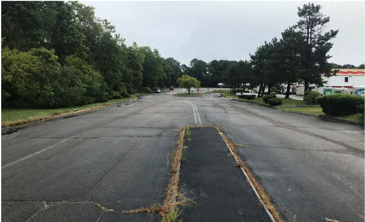
Photo #06: Looking west towards the project are with wetland buffer impacts to the left. Route 1 behind photographer
