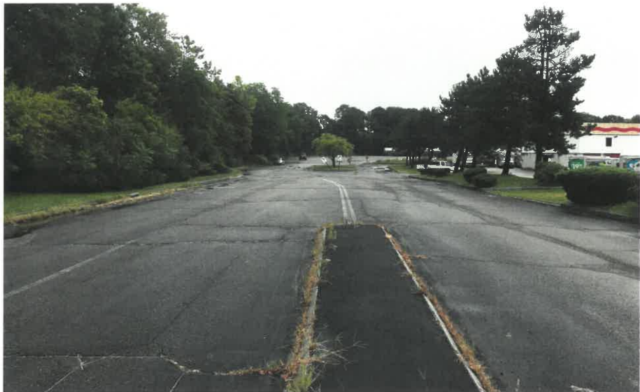
Photo #S6: Looking west towards the project are with wetland buffer impacts to the left. Route 1 behind photographer
