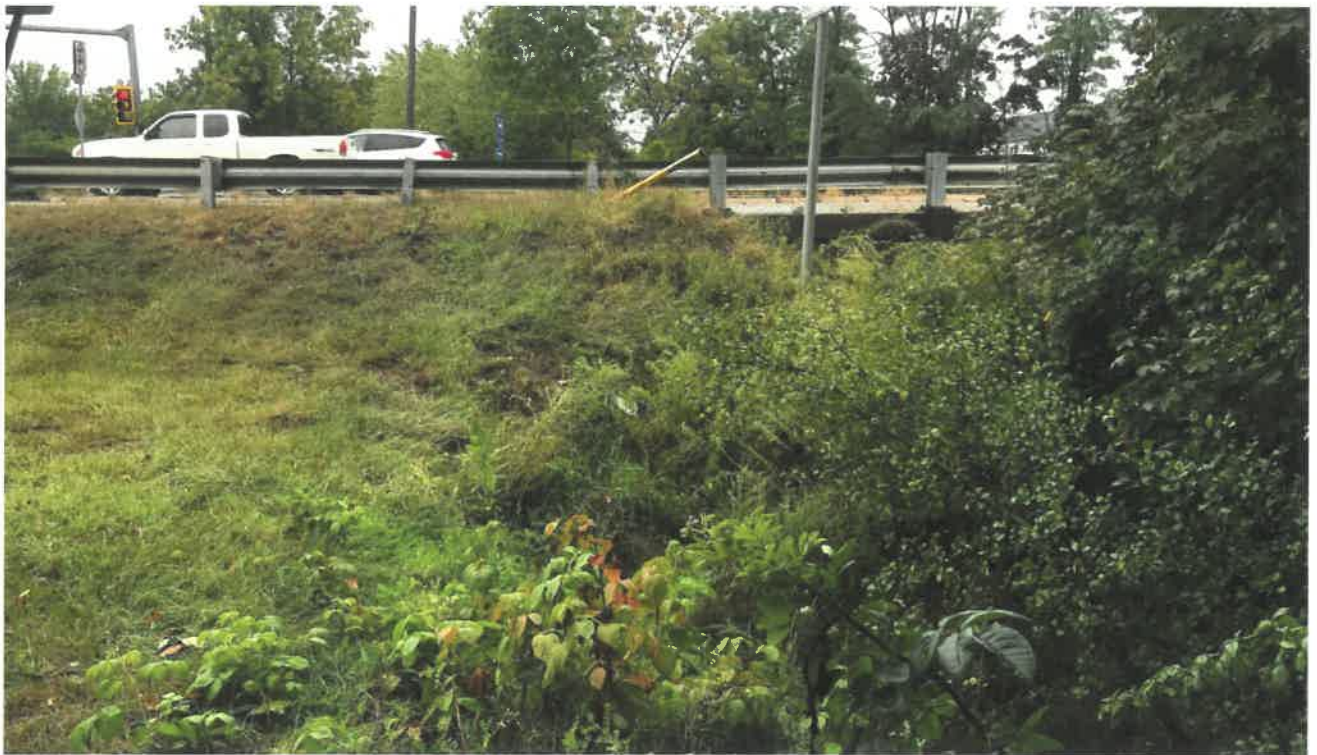
Photo I2: Impact area #1. Looking toward Route 1.
