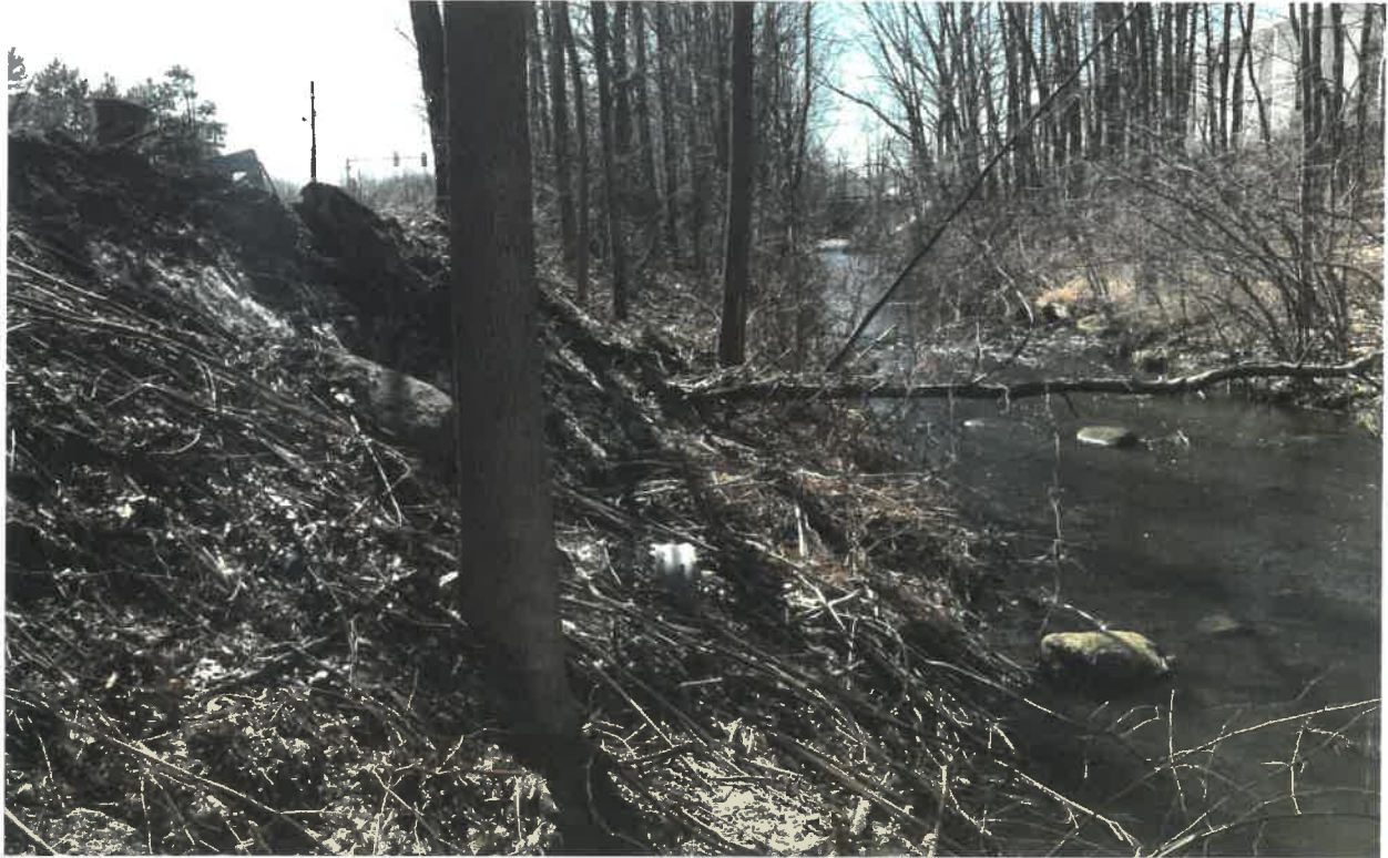
Photo I3: Looking towards Route 1 along the bank at impact area #2
