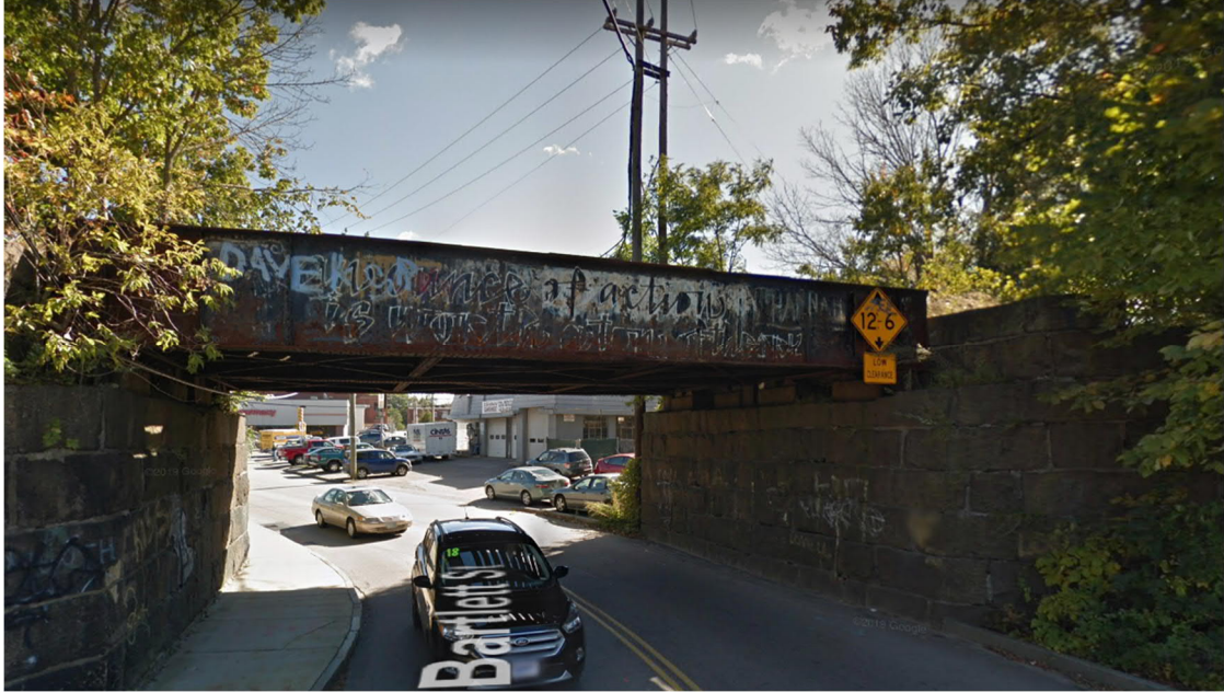
Bartlett Street looking south through the railroad overpass toward Islington Street – Low Clearance 12'6"
