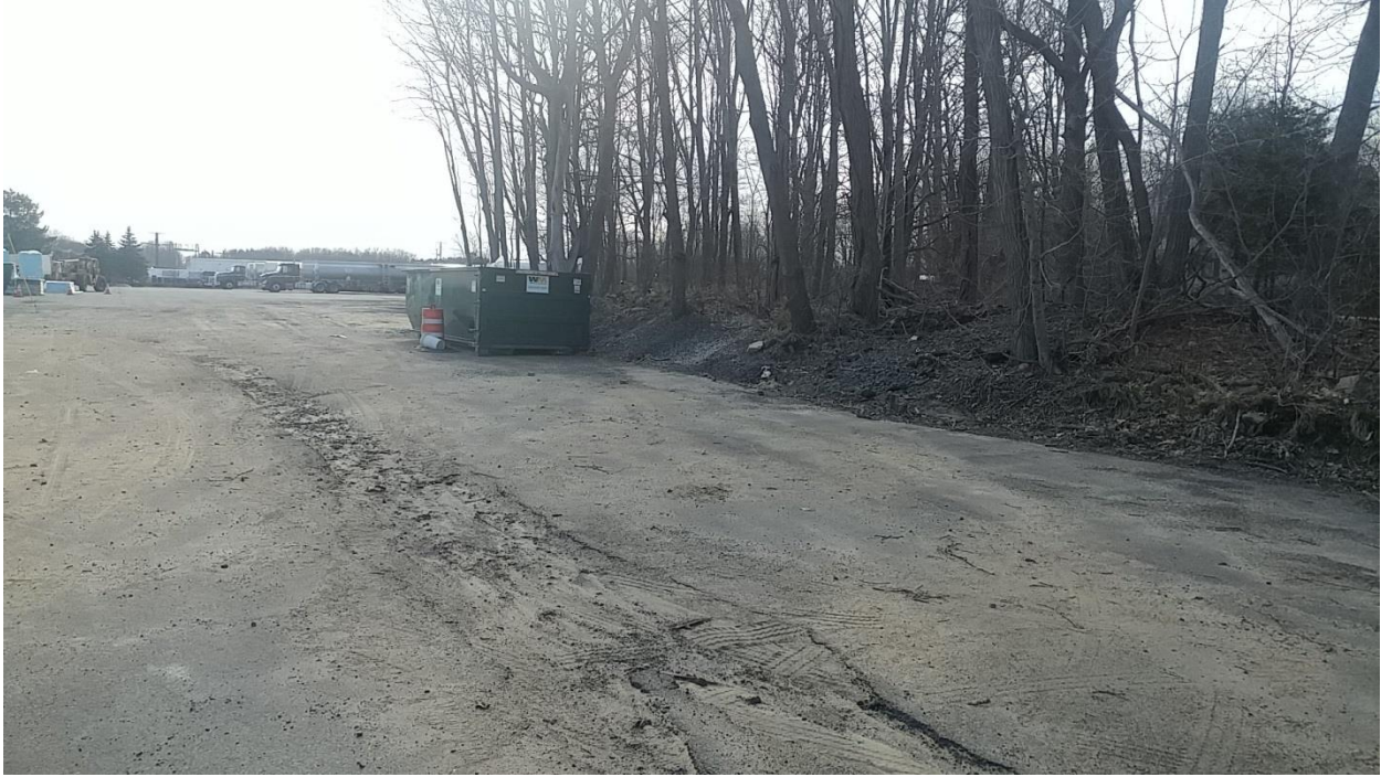
Photo 15 Access road off Cate Street looing west
