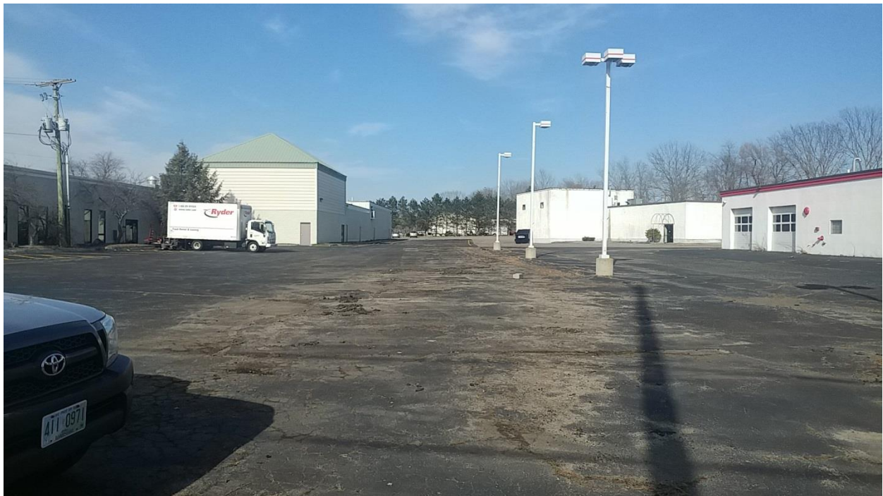
Photo 2 Rear of Frank Jones Center looking northeast
