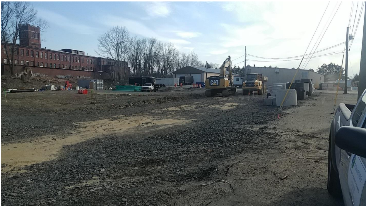
Photo 16 Current construction south of Cate Street looing southwest
