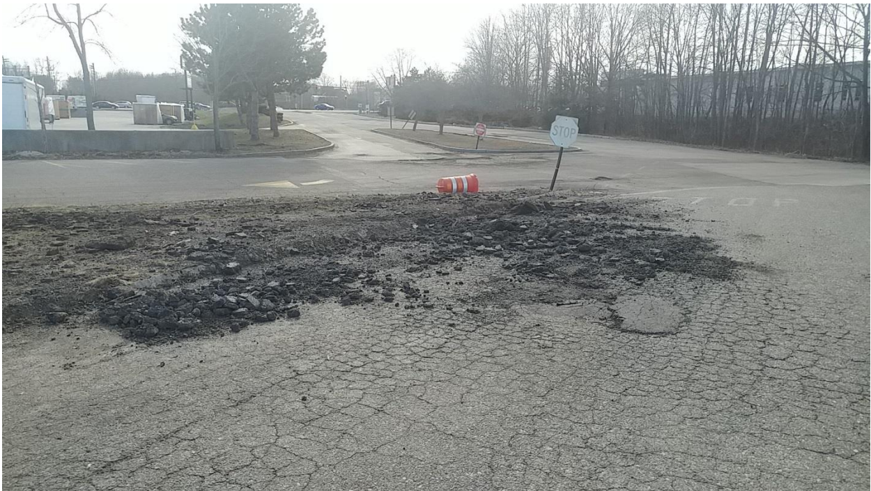
Photo 10 Looking west on Borthwick Ave towards Route 1
