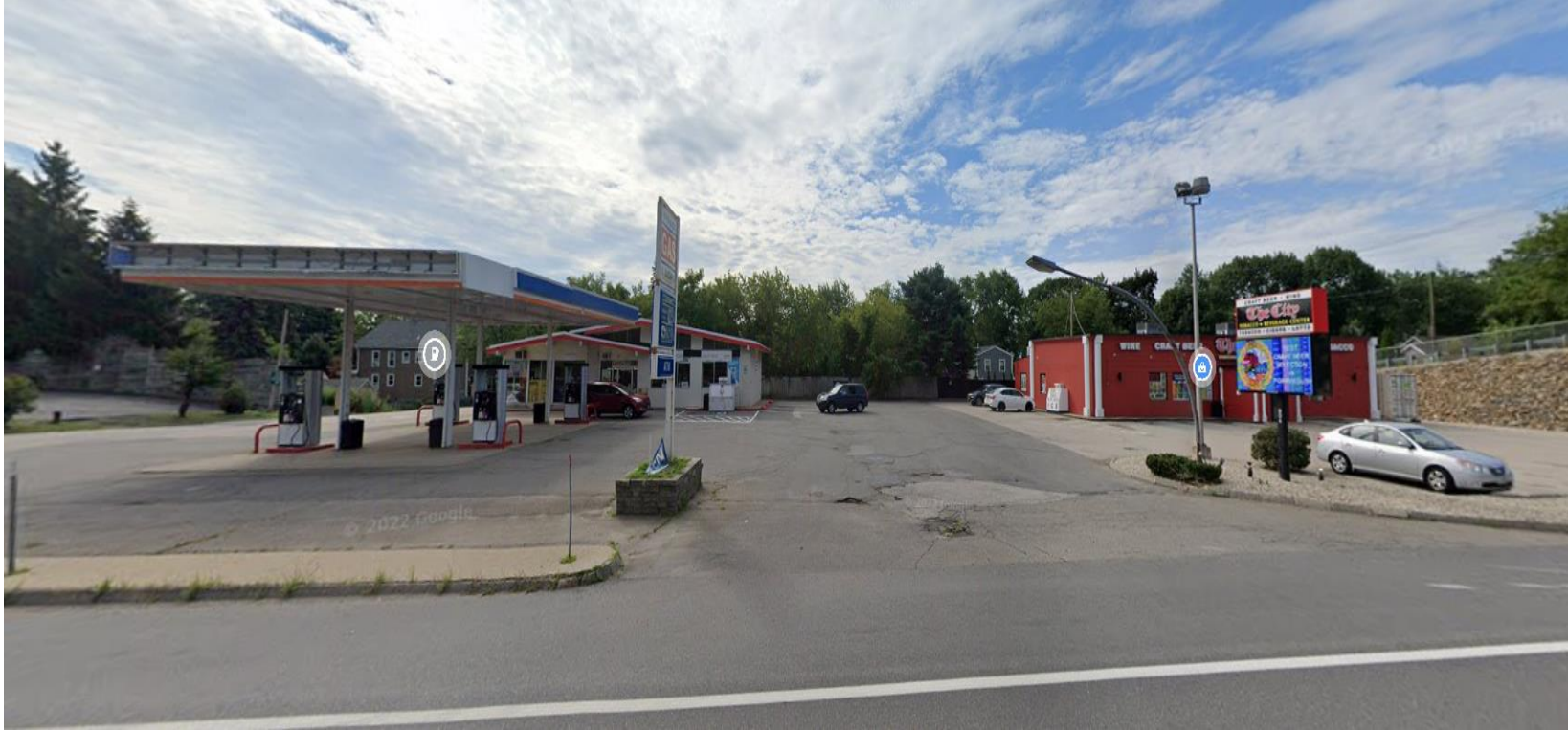
Photo 2: Front view 822 & 806 Rte 1 Bypass
