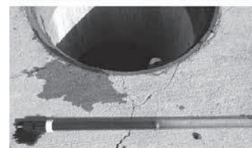
Inspection Utilizing Sediment Probe
