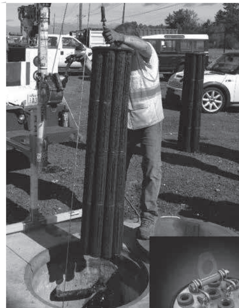
Cartridge Removal & Lifting Device
