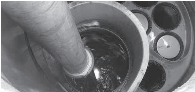
Vacuuming Sump Through MAW
