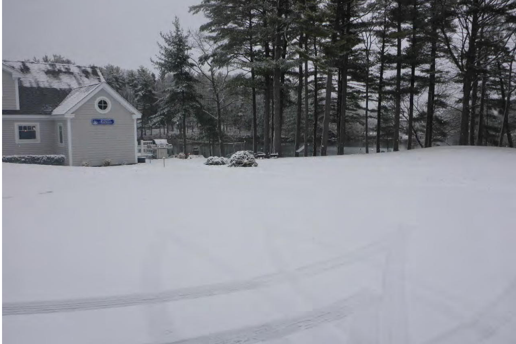
Photo 4: Facing north at 6 Sagamore Grove. Proposed location within the 100' TBZ for piping and grinder pump in existing maintained lawn. Sagamore Creek is seen in the background.
