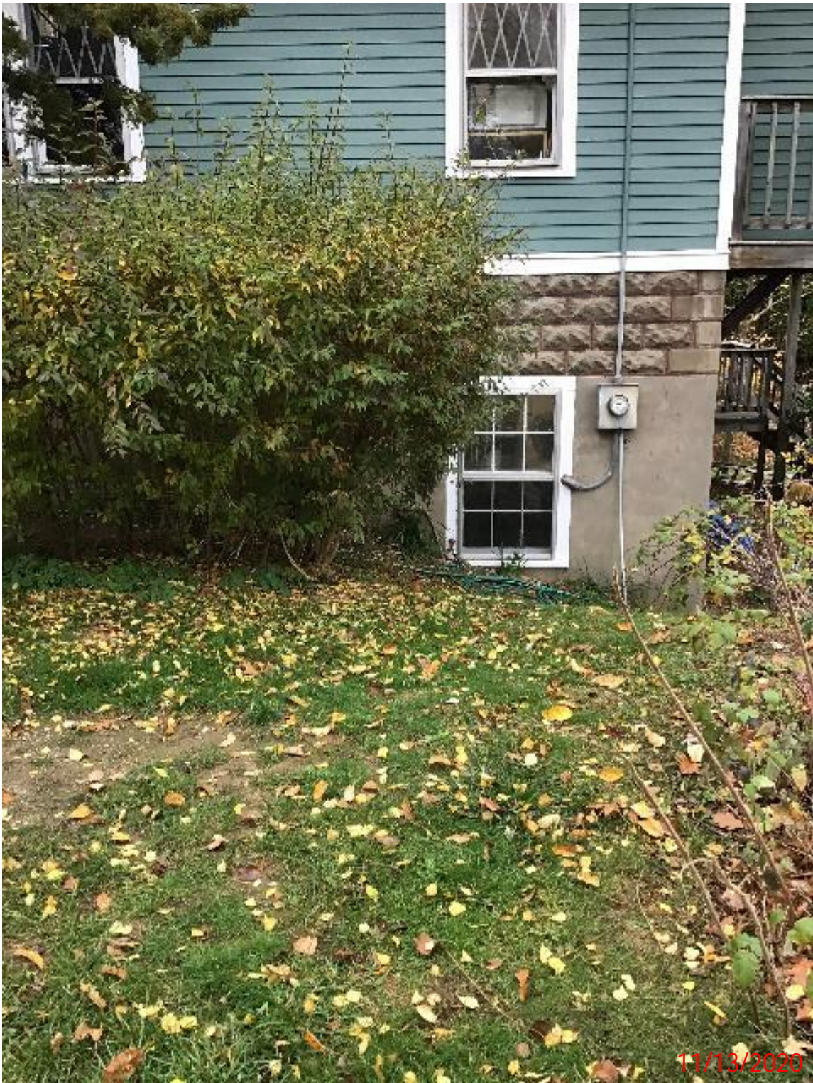
Photo 6: View of the South corner of 14 Shaw Road facing Northeast
