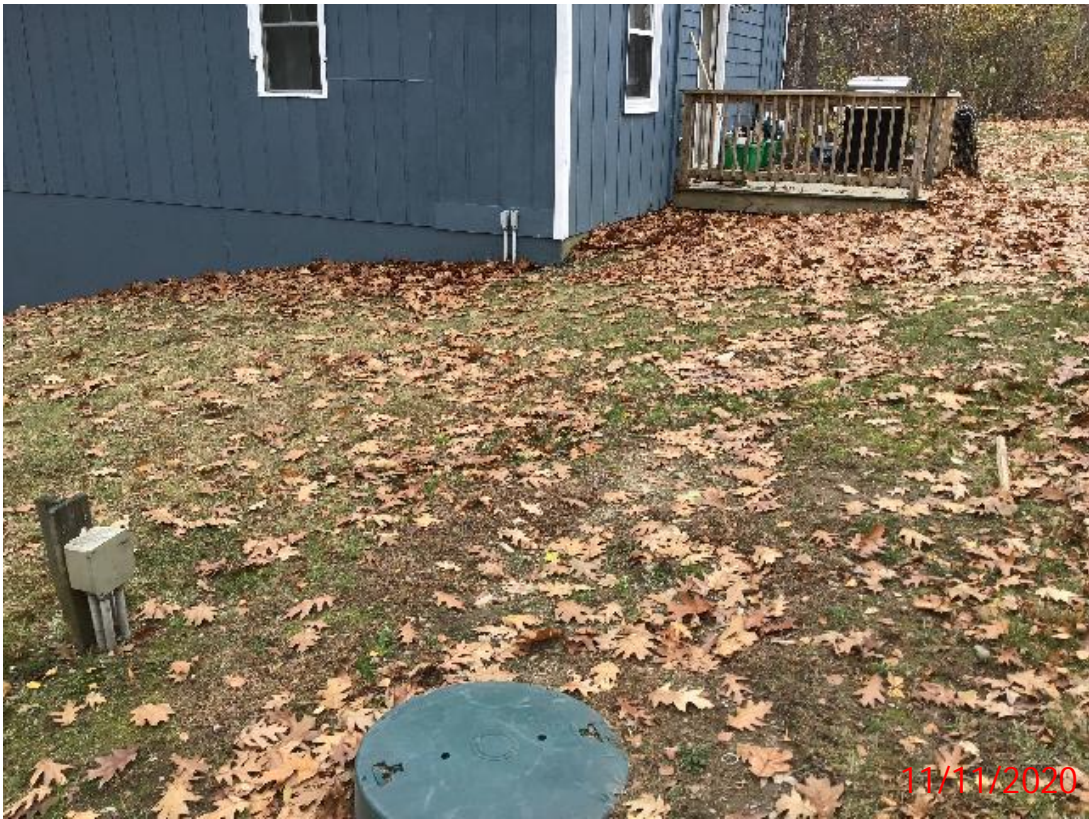
Photo 18: View of 913 Sagamore Avenue sewer lateral location, facing Southwest
