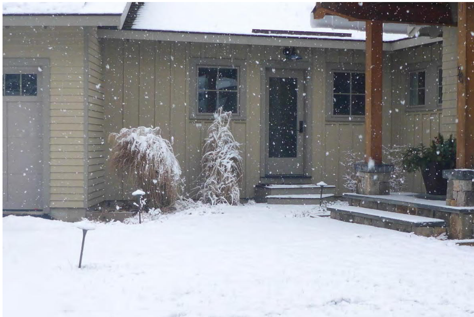
Photo 12: Facing east at 36 Shaw Road. Proposed location of piping and grinder pump in existing walkway and maintained yard within the 100' TBZ and 75' of salt marsh.
