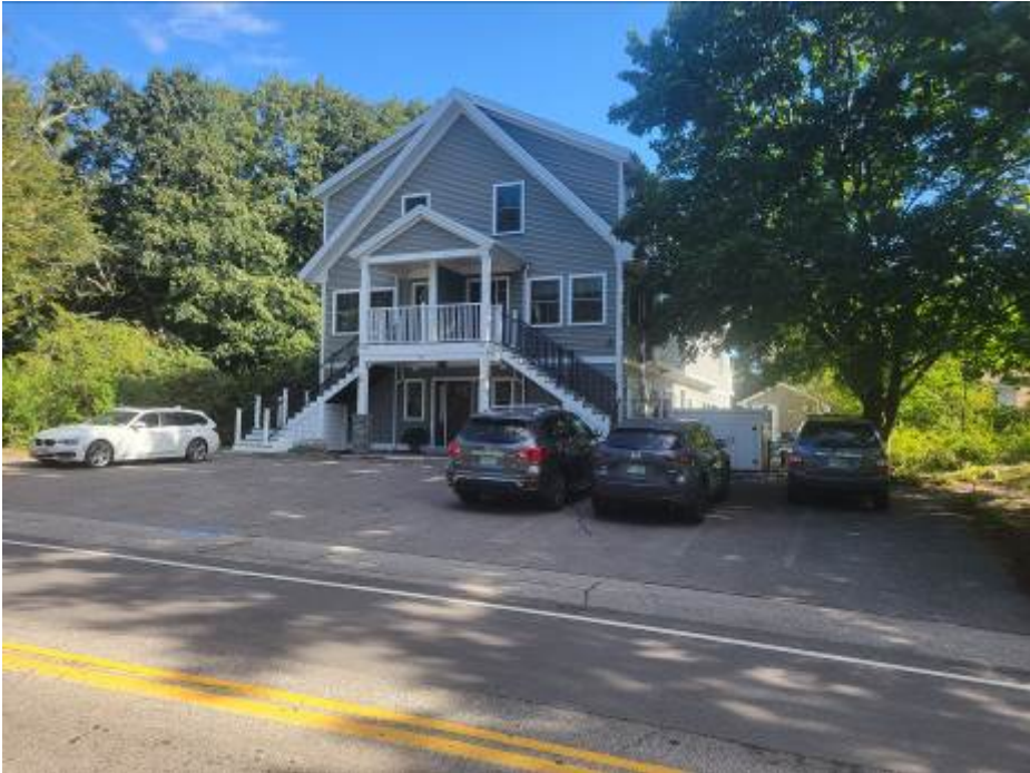
View of 792-796 Sagamore Avenue – Neighborhood Development Looking Northeast from Sagamore Avenue - (9/2023)
