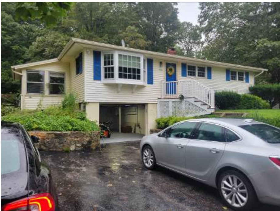
Front of the Subject Property Looking Southeast from Sagamore Avenue - (9/2023)
