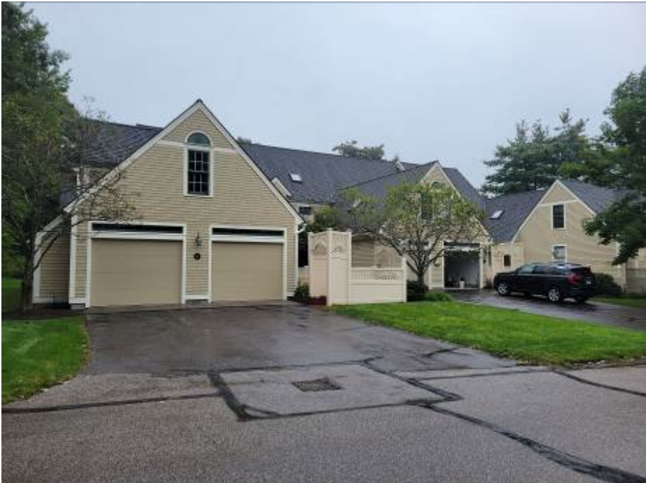
View of Tidewatch Condominium development – Typical Townhouse Building Looking East - (9/2023)
