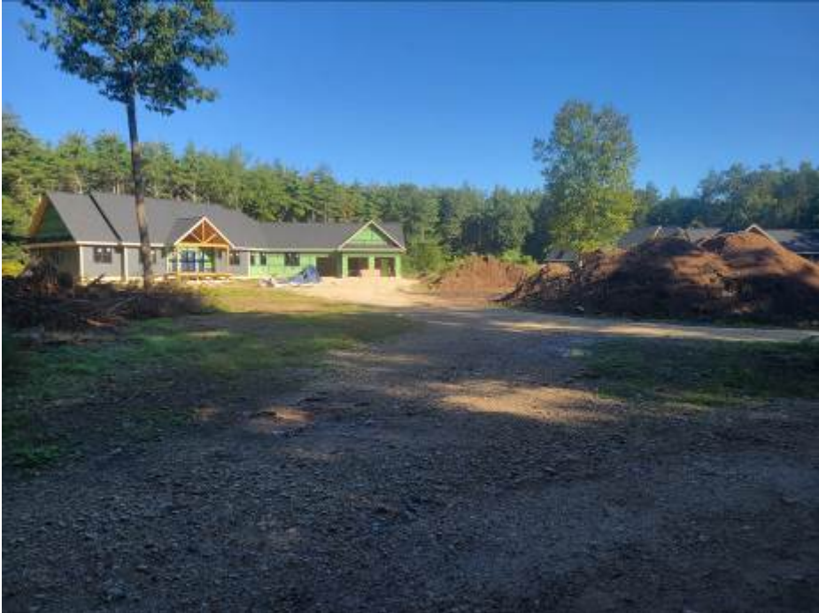
View of 400 Guld Road, Dover, NH – Multiple Residence Development Looking Northwest from Entry Drive - (9/2023)
