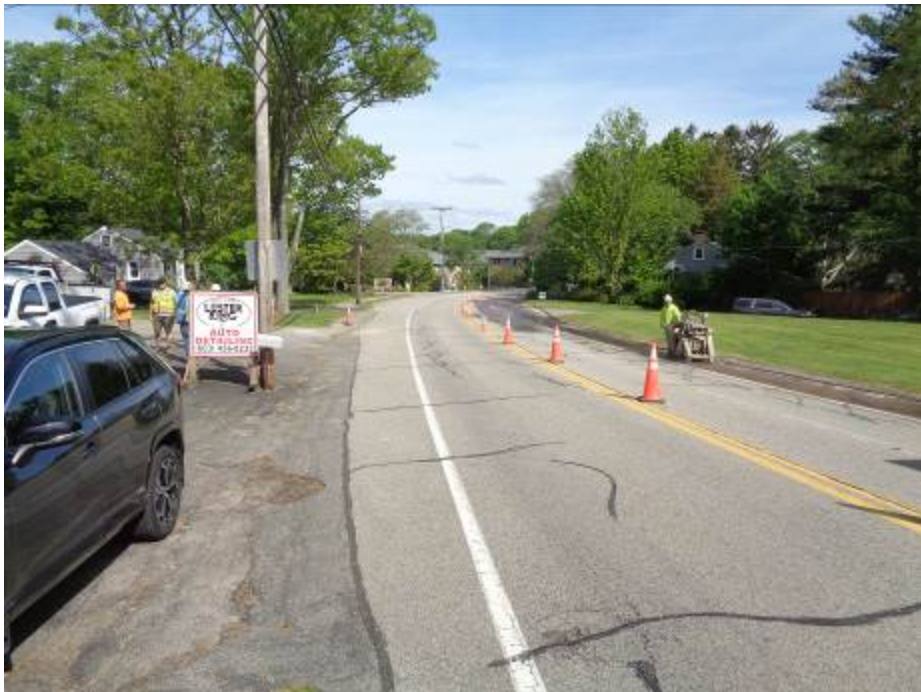
Street Scene - Front of the Subject Property Looking Southeast on Sagamore Avenue - (5/22)
