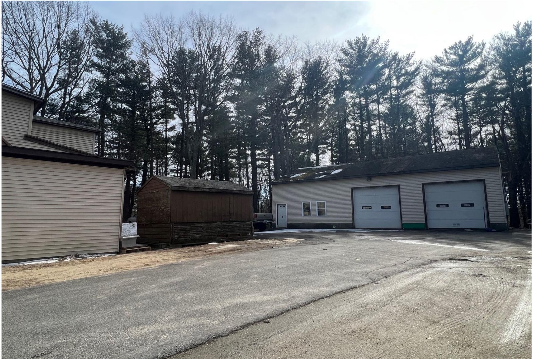
View of Service Garage and Shed
