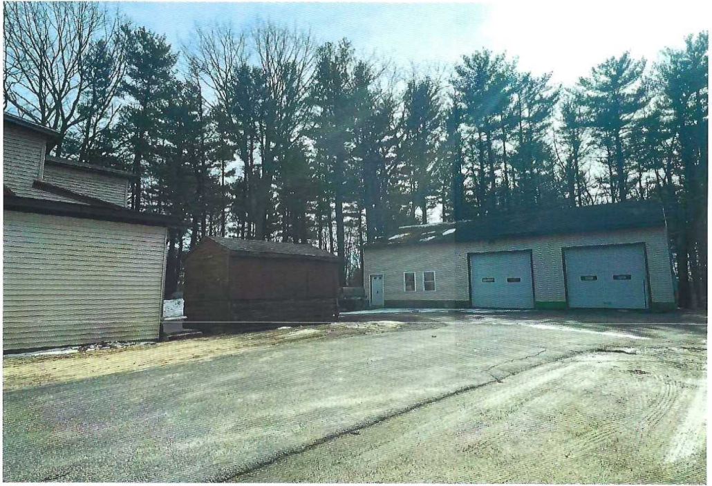
View of Service Garage and Shed
