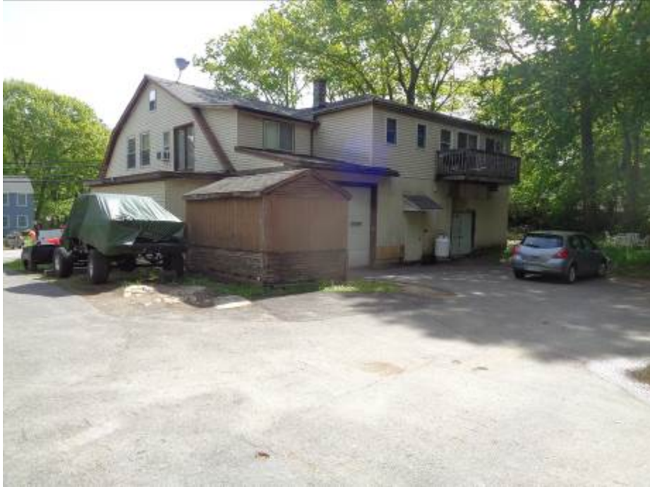
Subject Property – Rear of the Front Mixed-use Building Looking East from Rear Paved Area – (5/22)
