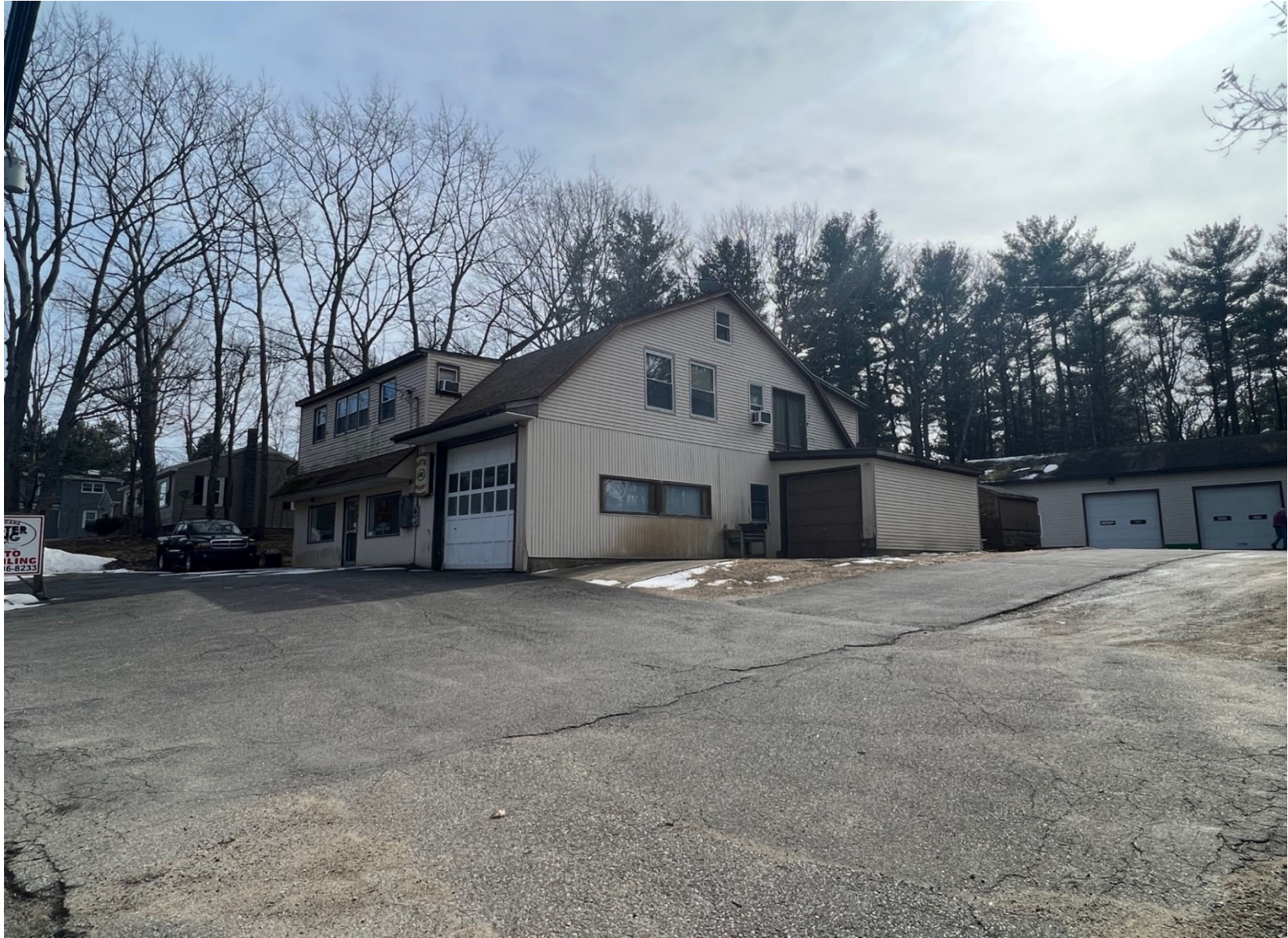
Side View of Property
