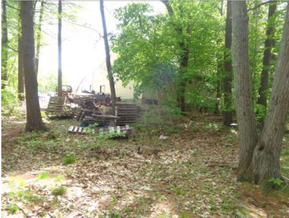
Subject Property – Rear of the Rear Garage Building Looking Northeast from Rear Wooded Area – (5/22)
