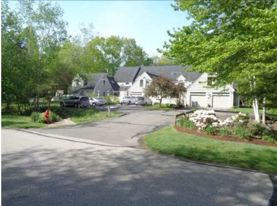
View of Typical Tidewatch Condominium Building Looking South from Access Road - (5/22)
