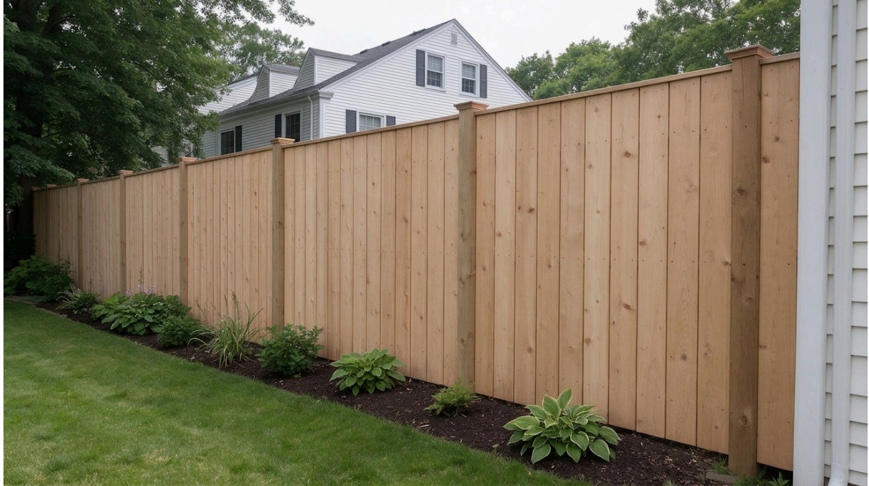
Image illustrating the general style of the 5-foot high cedar colonial replacement fence that would be installed.
