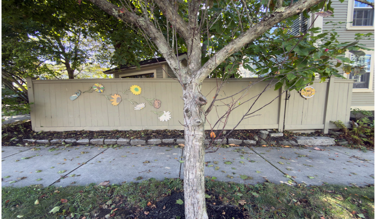
Existing 5-Foot cedar fence along our property frontage on the left side of our house.
