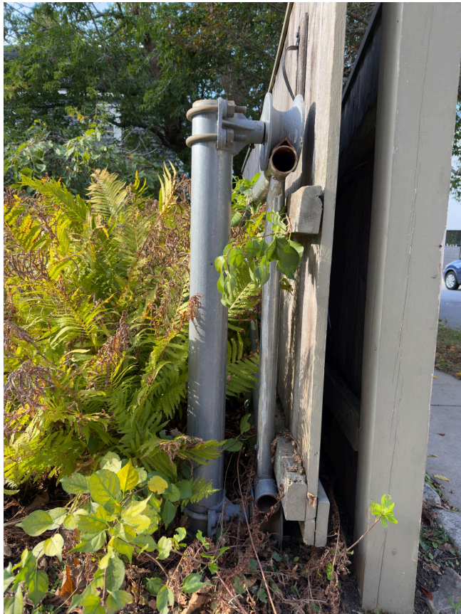
Steel sliding gate operating assembly for 5-foot cedar wooden gate.
