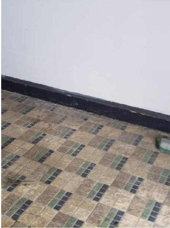
Figure 17 – Vestibule floor gap below baseboard
