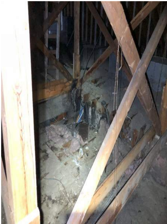
Figure 7 – Cupola tower and ceiling joists fire damage
