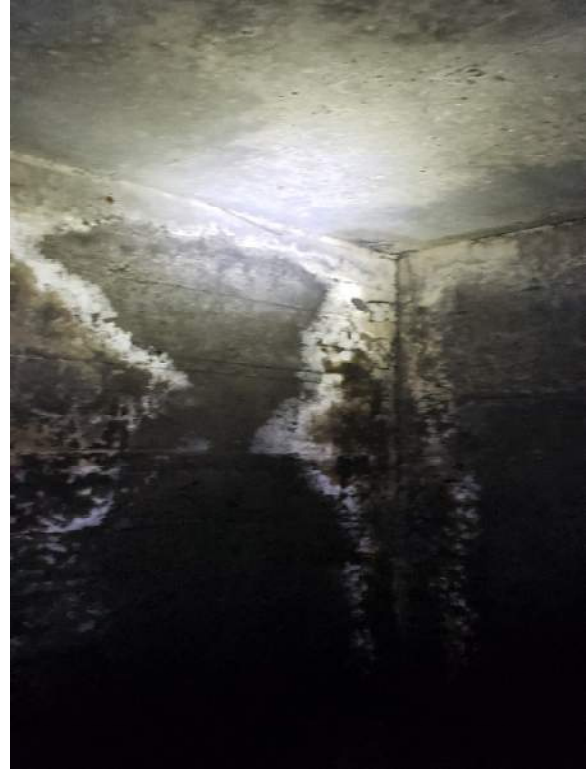
Figure 22 – Basement concrete wall efflorescence
