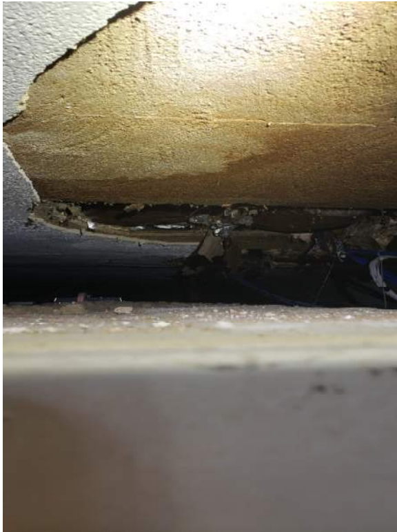
Figure 1 – Water damage ceiling
