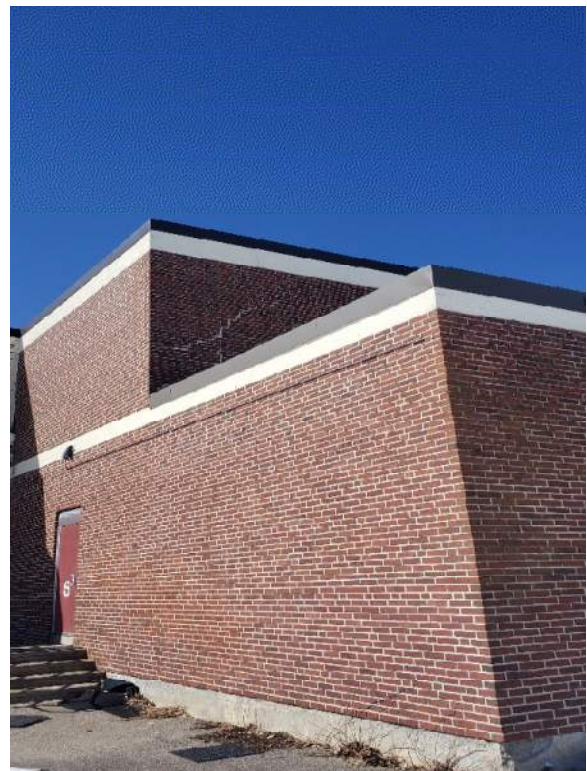
Figure 28 – Exterior vertical stepped masonry crack at gym
