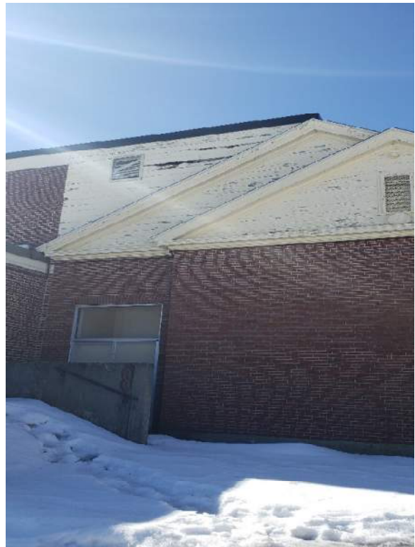
Figure 8 – Exterior wood siding and trim rot
