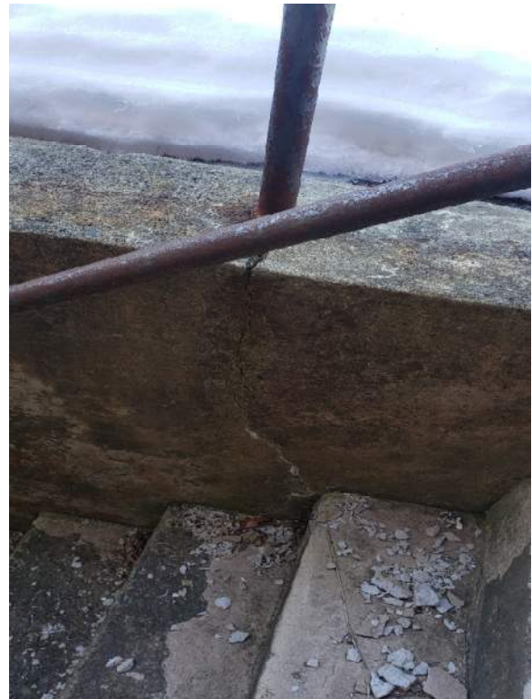
Figure 24 – Exterior stairway vertical wall crack and tread damage
