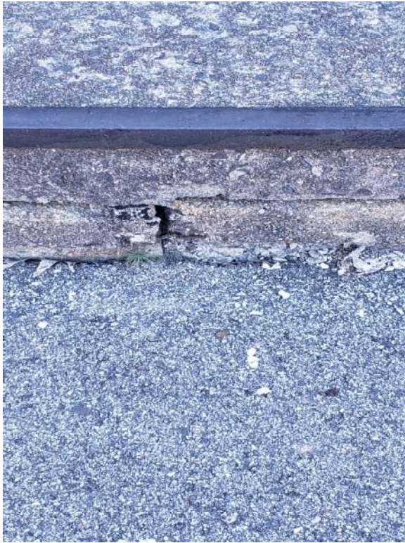
Figure 25 – Exterior coal chute failed concrete
