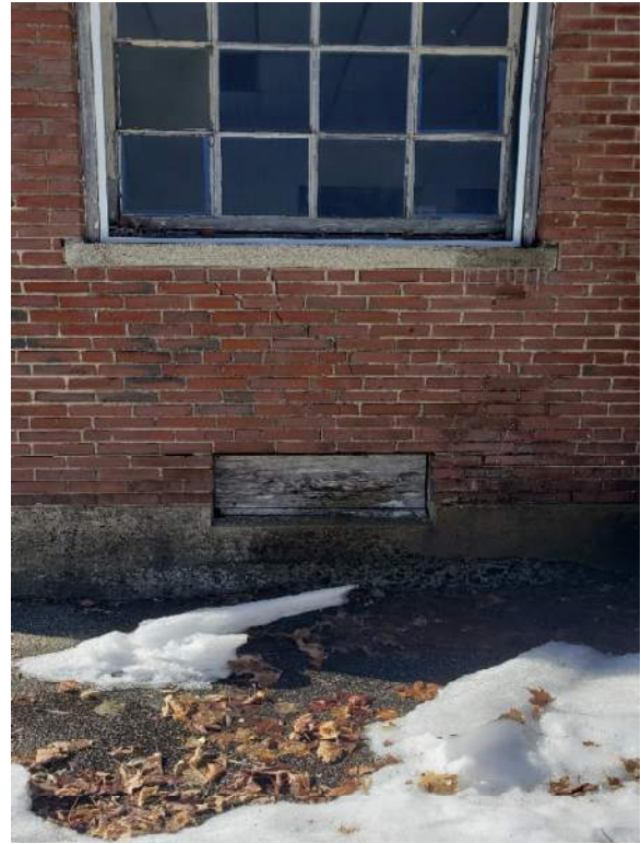
Figure 10 – Exterior masonry mortar loss and water damage
