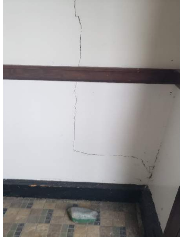
Figure 18 – Vestibule wall vertical stepped cracks
