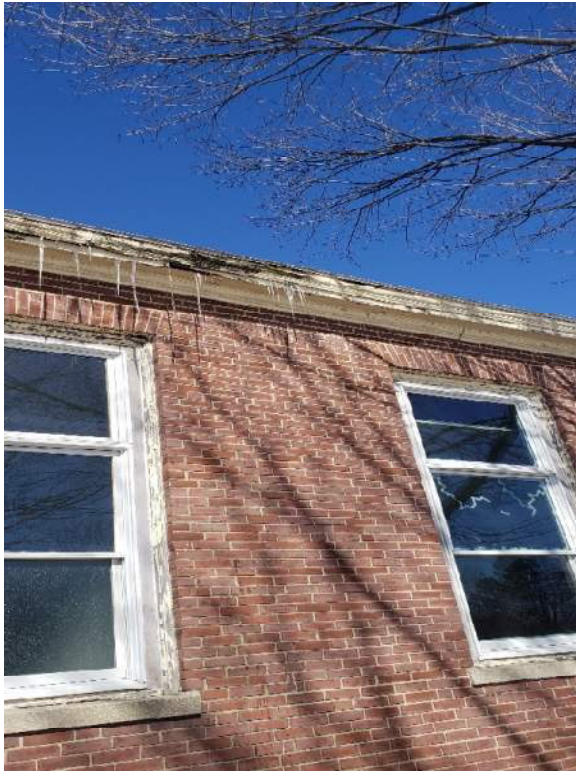
Figure 13 – Exterior eave trim wood rot and water damage
