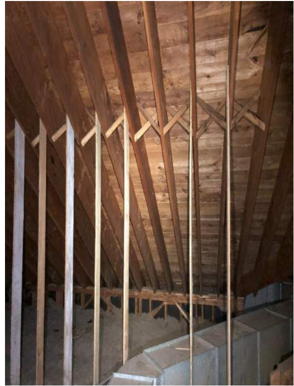
Figure 26 – Ceiling joist hangers at roof rafters
