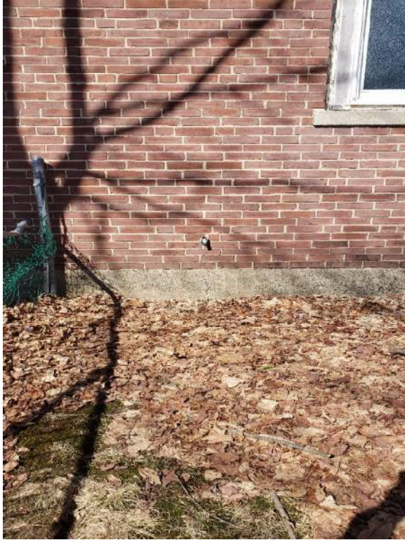
Figure 21 – Exterior foundation vertical crack below spigot
