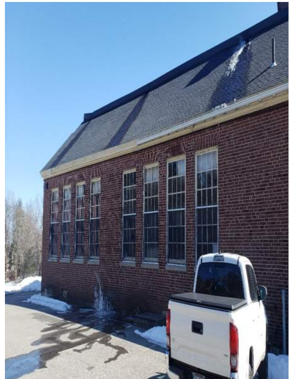
Figure 16 – Roof drainage away from scuppers
