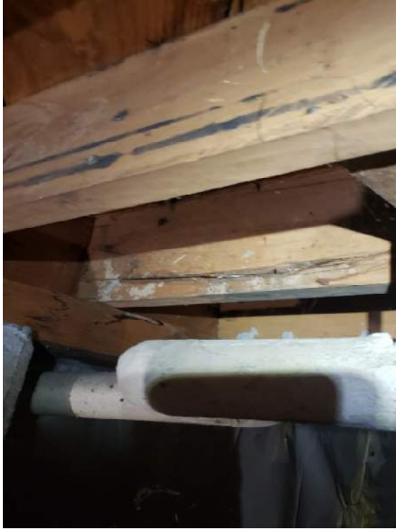
Figure 5 – Floor joist split end
