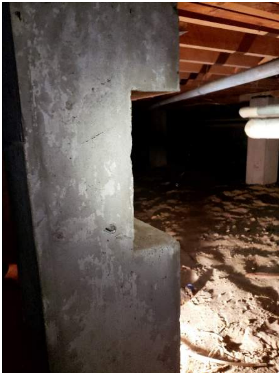
Figure 19 – Crawl space pier notch
