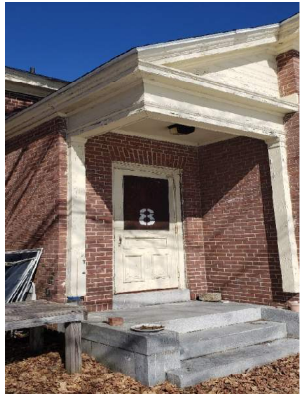
Figure 12 – Missing wood post at corner
