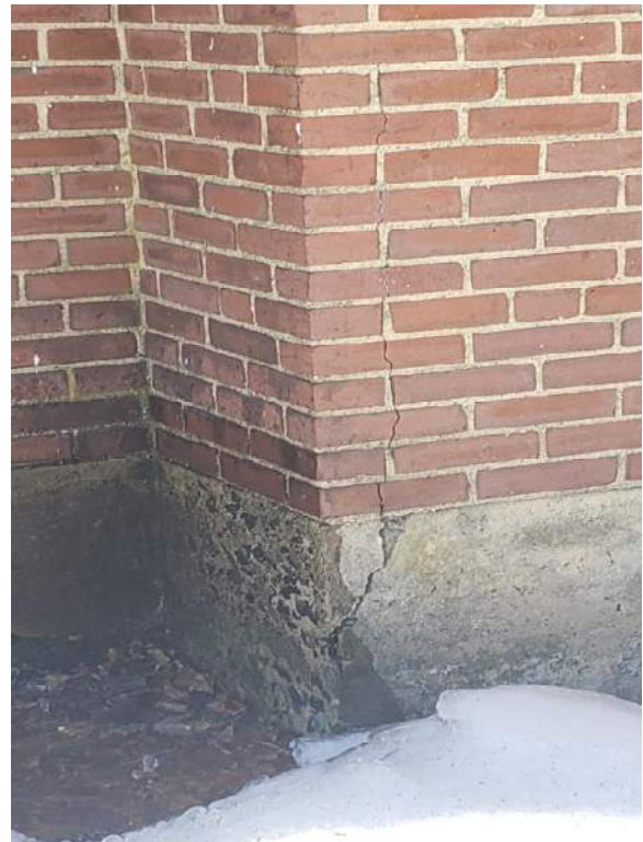
Figure 20 – Exterior foundation and masonry vertical crack
