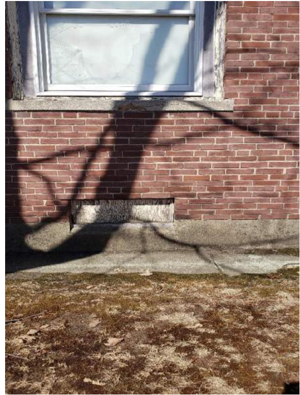
Figure 14 – Exterior concrete sill damage and broken window
