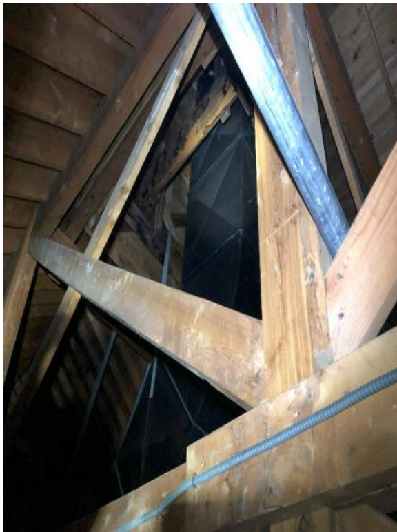
Figure 3 – Water-stained cupola tower framing
