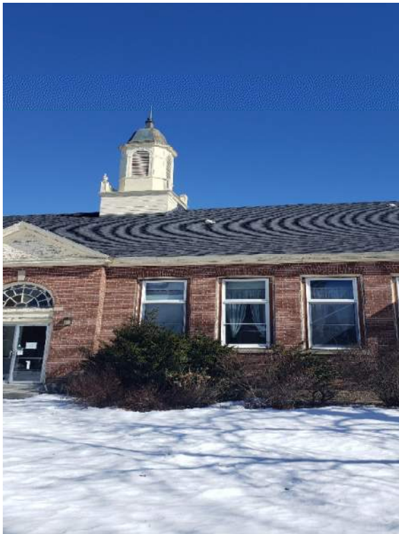
Figure 15 – Cupola railing and finials missing
