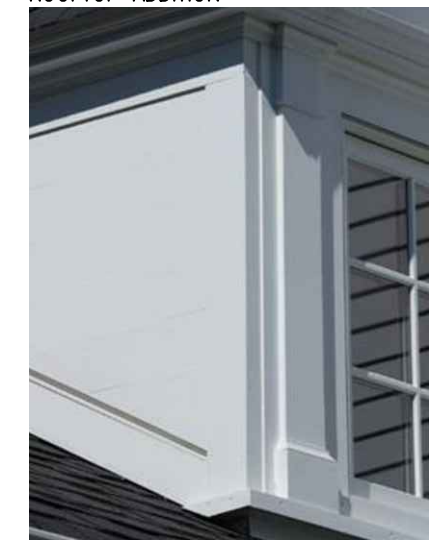
SHIPLAP BORAL SIDING AT ROOFTOP ADDITION
