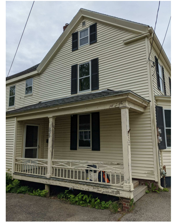
PARTIAL VIEW FROM NORTH ELEVATION
