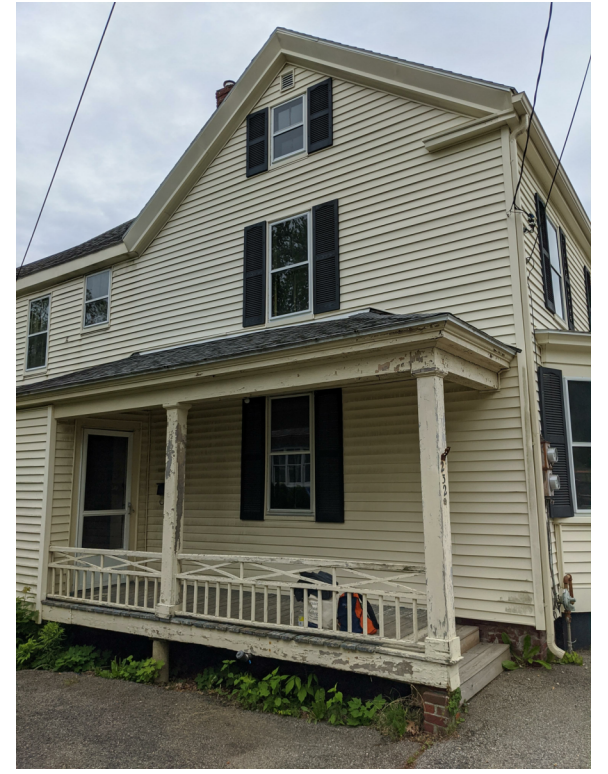
PARTIAL VIEW FROM NORTH ELEVATION
