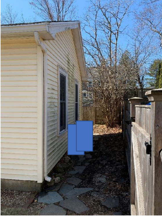
Rear of property showing approximate location of heat pump units, below fence line.
