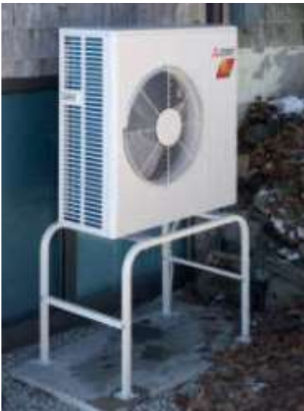
Example heat pump outdoor unit, 22" high with 24" inch stand. Total height 46" or 3' 10".
