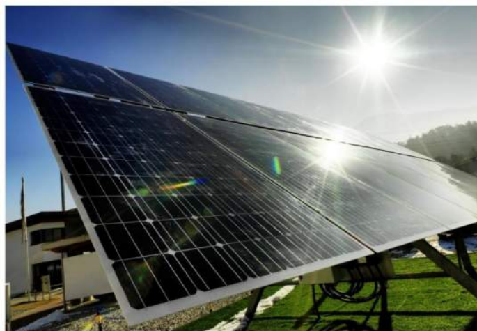
Solar panel showing solar glare
